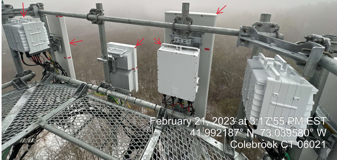
Alpha Sector: (3) New Antennas & (2) New RRHs On Existing Mounting Platform
