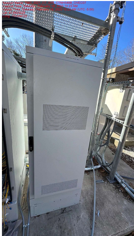
New Battery Cabinet Mounted To Existing Concrete Pad
