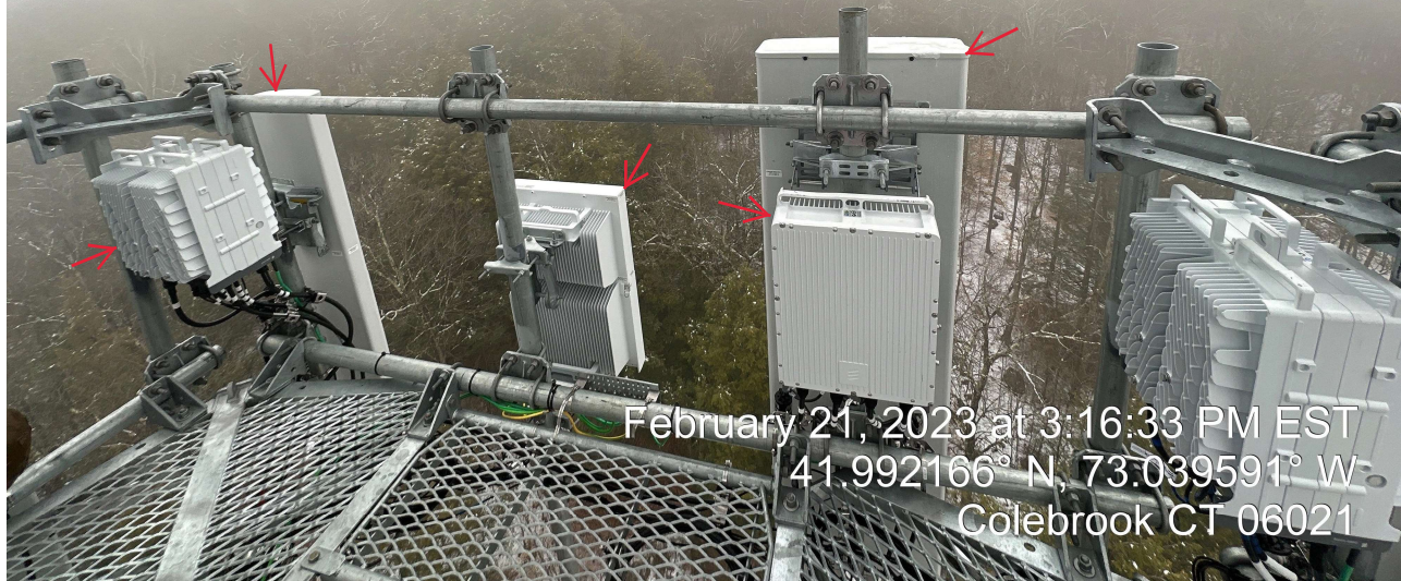
Beta Sector: (3) New Antennas & (2) New RRHs On Existing Mounting Platform
