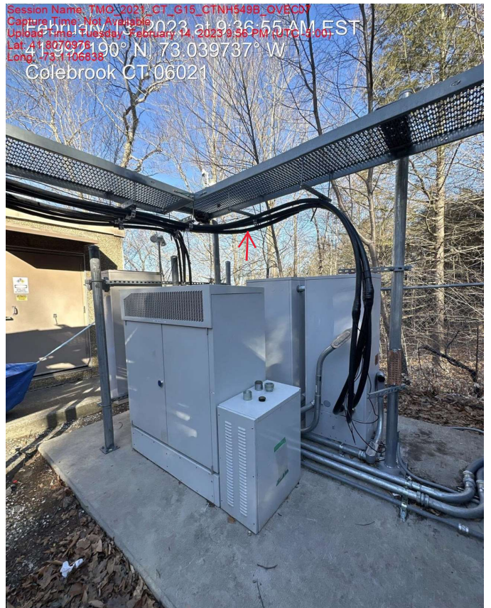
(3) New Signal Cables Run Along Existing Cable Path
