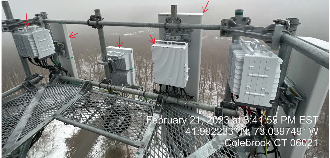
Delta Sector: (3) New Antennas & (2) New RRHs On Existing Mounting Platform
