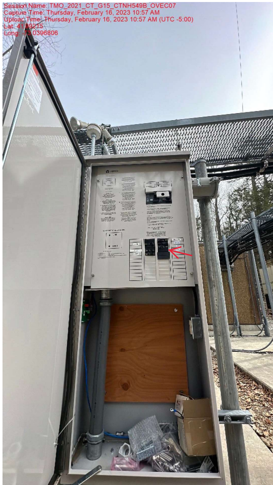
New Cabinets Tied Into Existing Electric Panel
