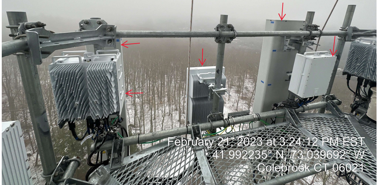
Gamma Sector: (3) New Antennas & (2) New RRHs On Existing Mounting Platform
