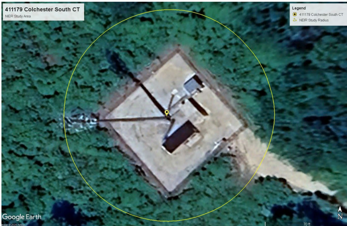
Aerial View of Site
