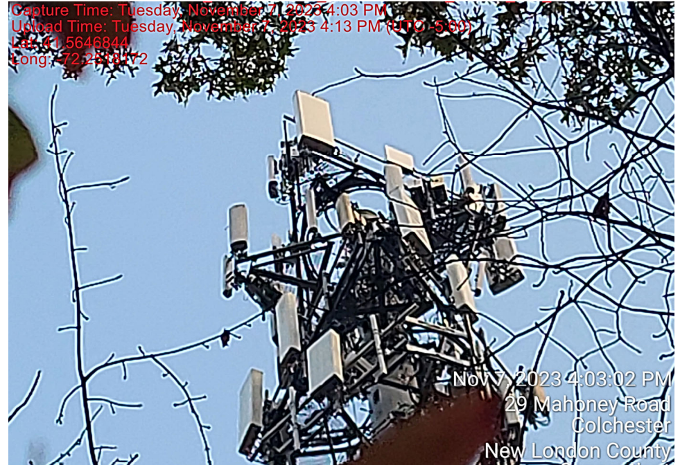
Beta sector antenna installation on existing sector frame
