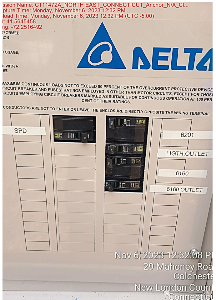
New breakers installed in existing PPC
