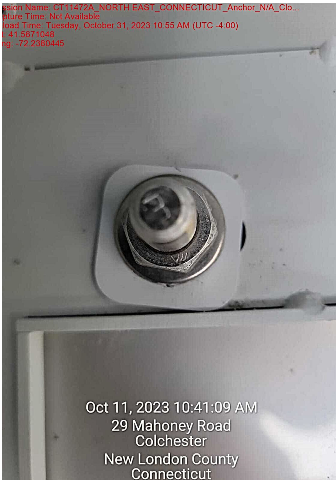
New anchor bolts installed at base of cabinet
