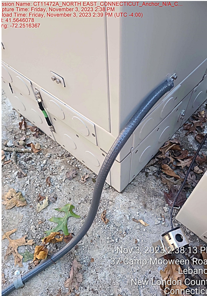
New ground connection installed at base of cabinet
