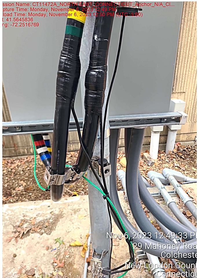
New slack box installed on new H-Frame
