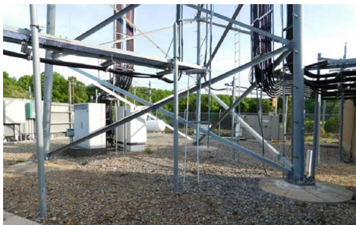
TOWER BASE/FOUNDATION PHOTO
