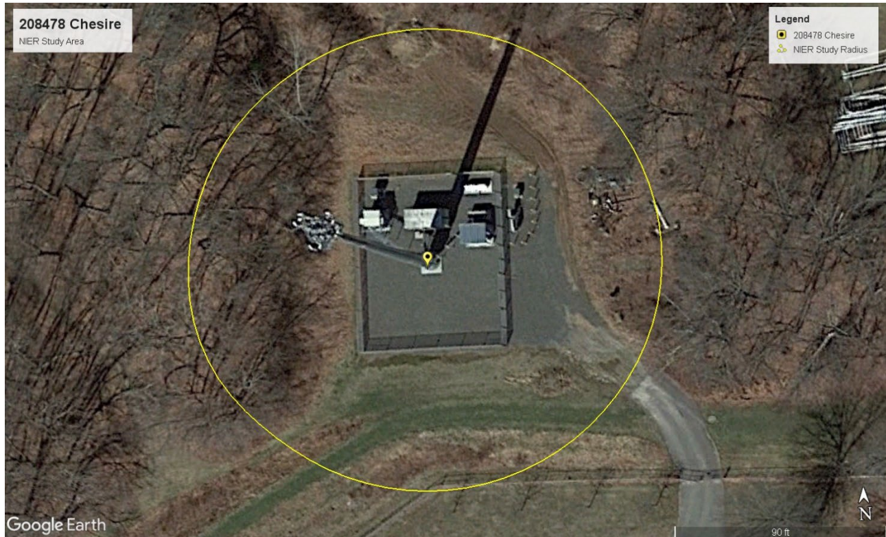
Aerial View of Site
