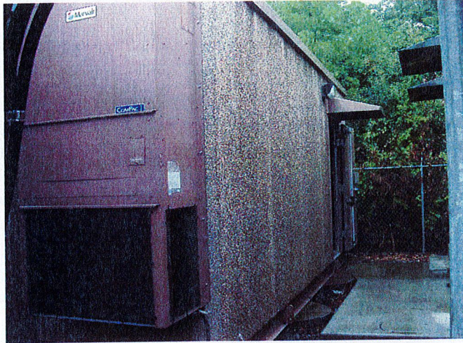
FORMER AT&T GROUND SHELTER
