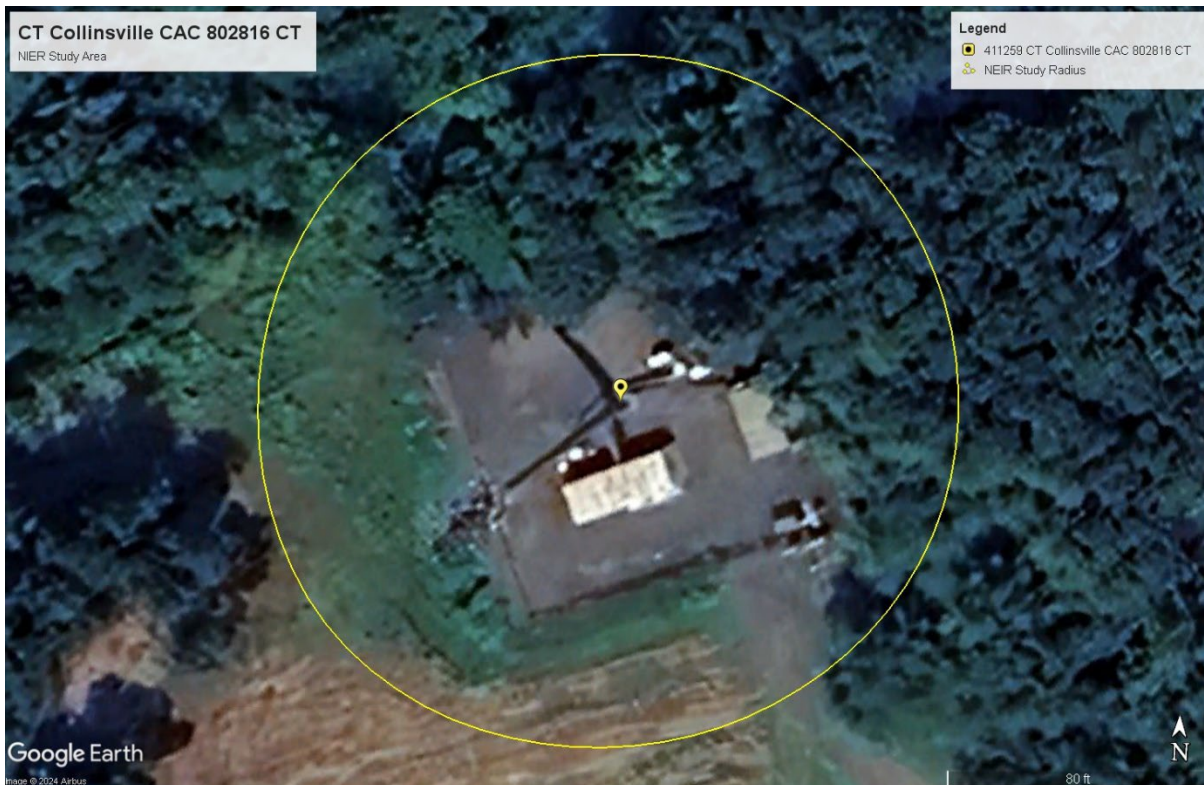
Aerial View of Site
