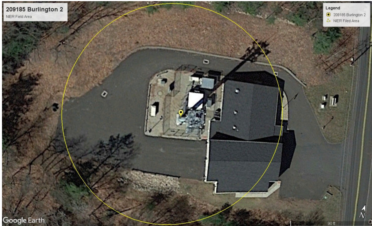
Aerial View of Site
