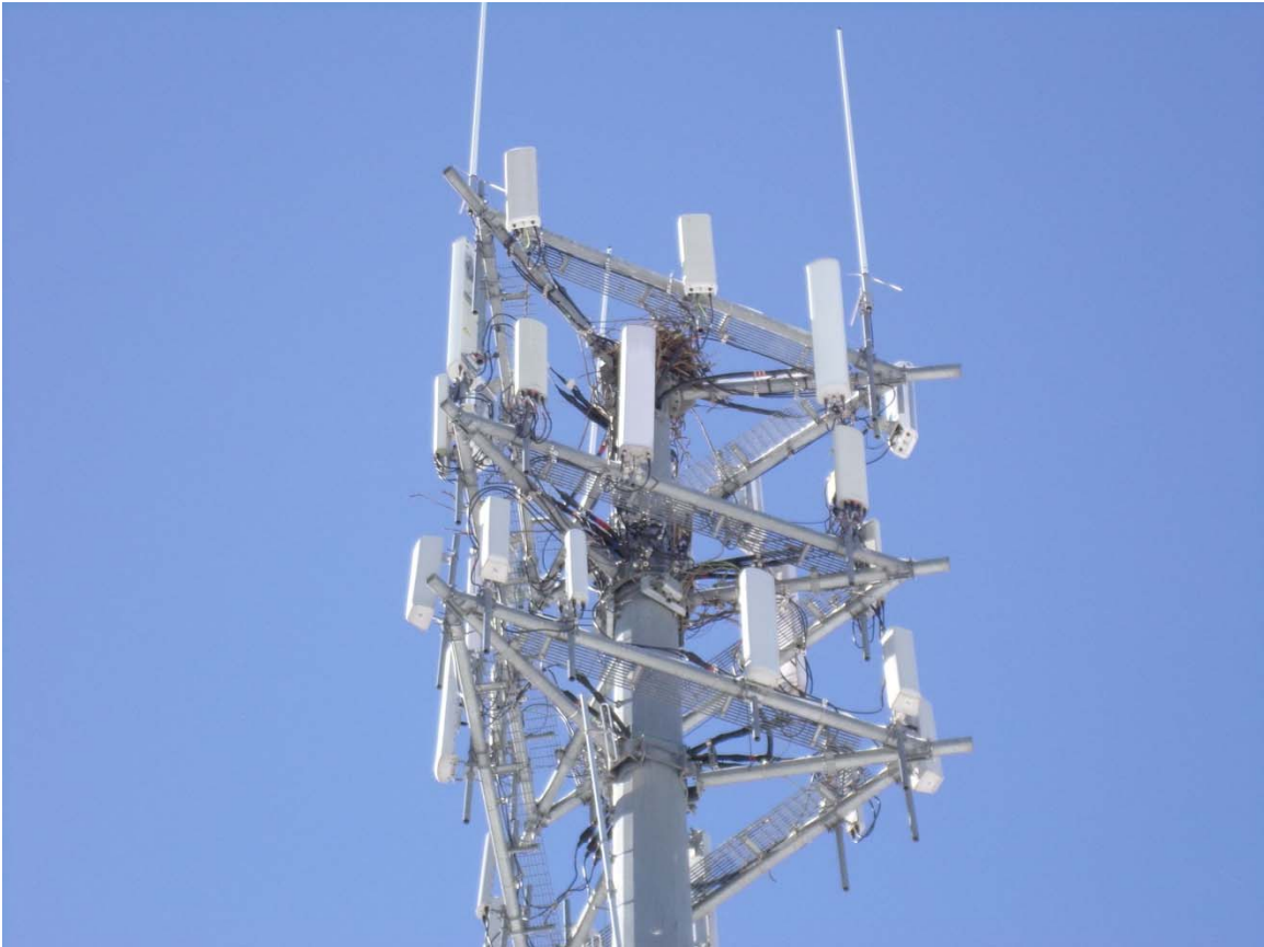
Photo 1: Photo illustrating the monopole with Appurtenances shown.
