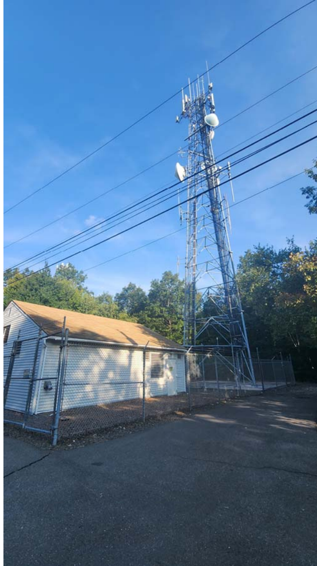
Figure 1: View of ES-004 South Mountain
