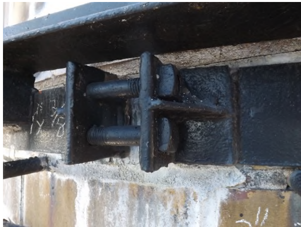
Existing Catwalk Assembly Connections
