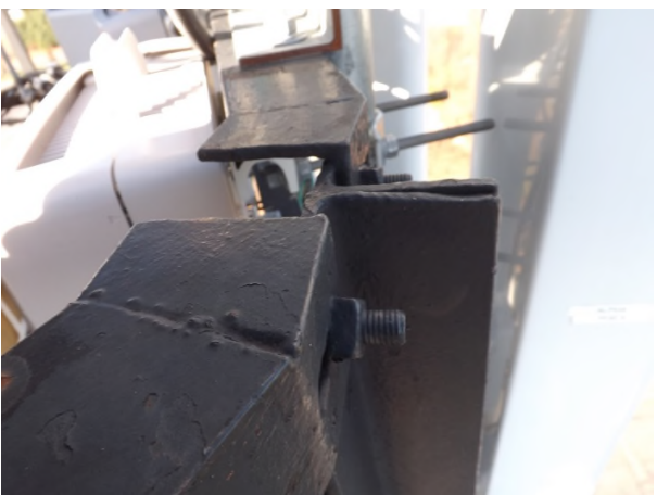
Existing Catwalk Assembly Connections
