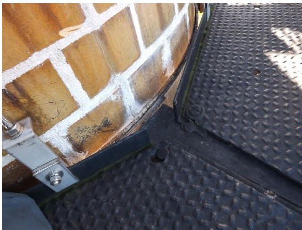
Existing Catwalk Assembly Connections
