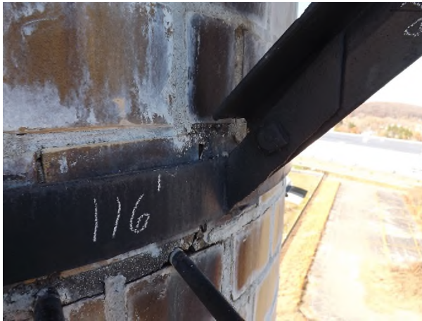
Existing Catwalk Assembly Connections
