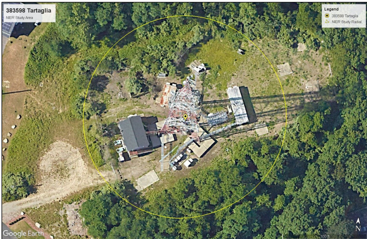
Aerial View of Site
