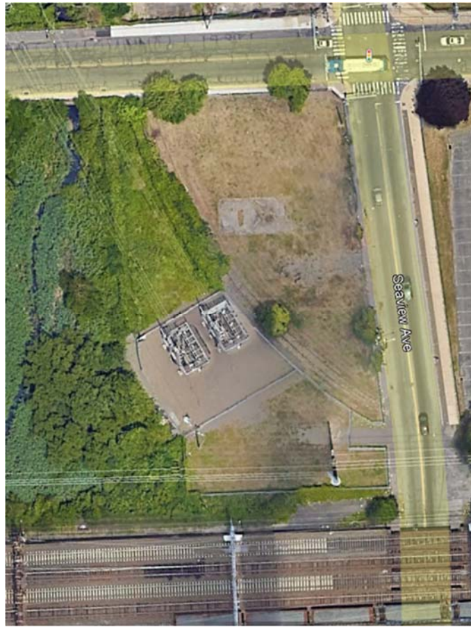
Existing Seaview Tap Substation Yard, Google maps, 2022
