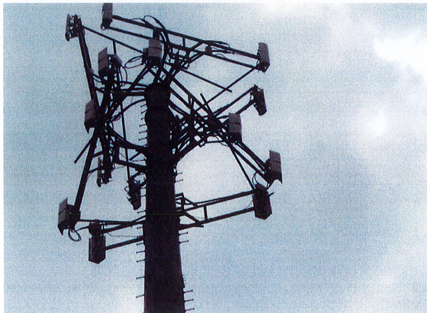
AT&T ARRAY REMOVED AT 165'
