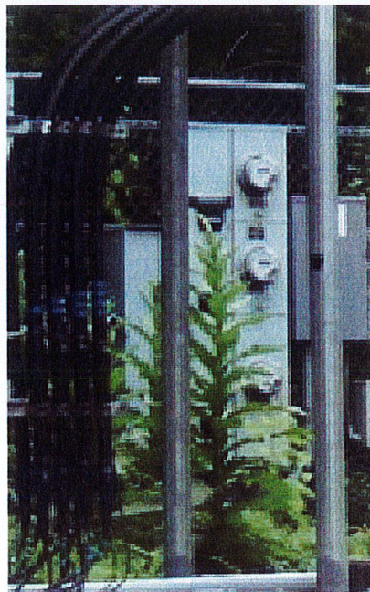
AT&T ELECTRICAL & TELEPHONE TO BE REMOVED
