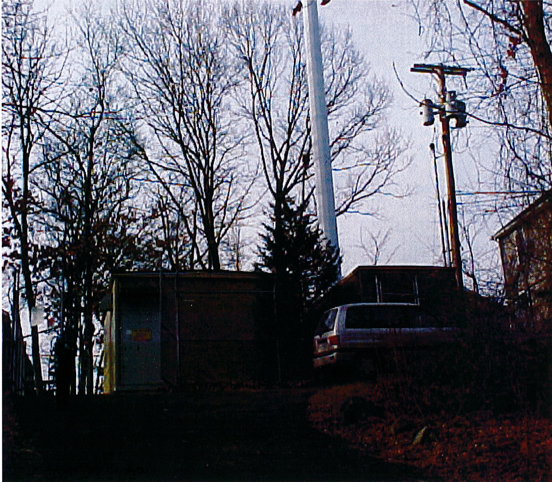
Figure 4. View of the controlled area enclosure for the Ox Hill monopole.
