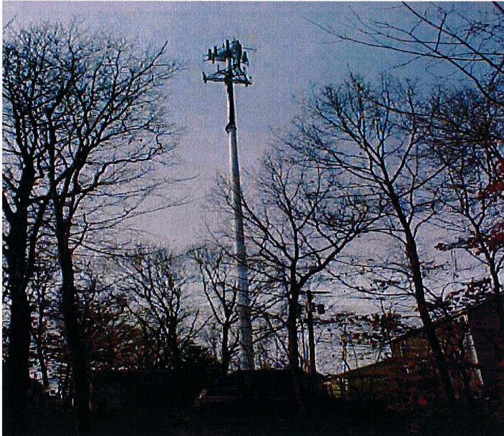
Figure 2. View of the Ox Hill monopole.
