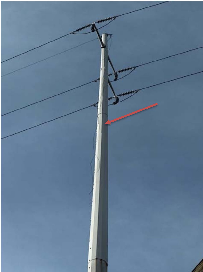
Picture 2 - Static hanging from atop Structure 775B
