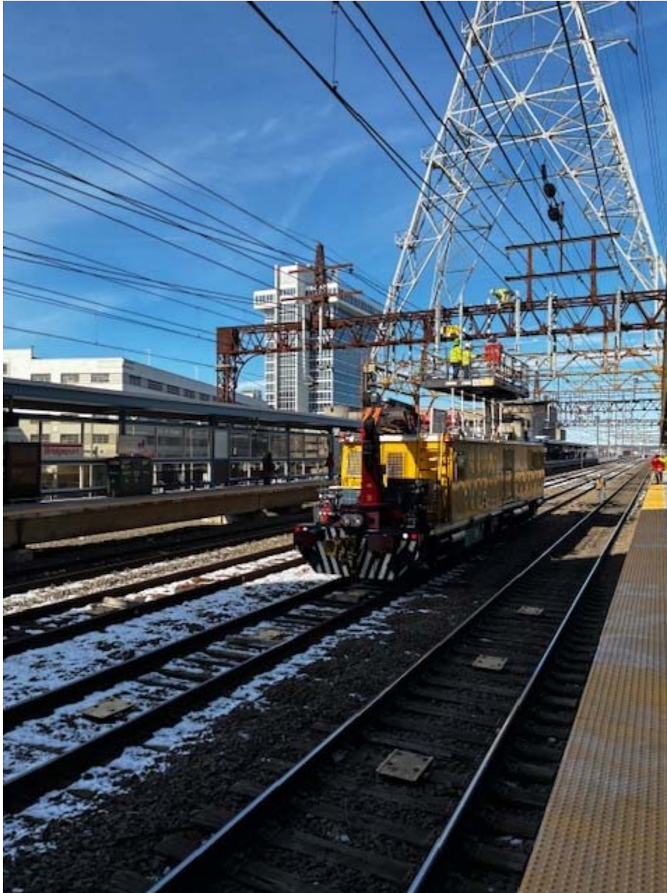
Picture 5 – MNR and UI crews working to remove UI static wire laying across MNR facilities.
