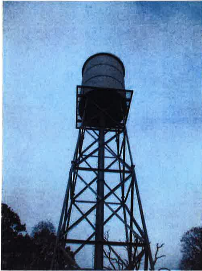
Photo 1: Sample photo illustrating existing water tank.
