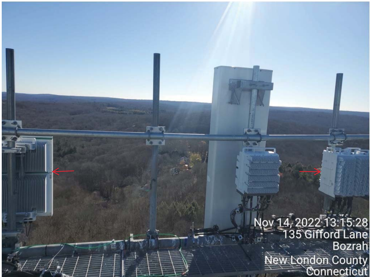
Beta Sector: (1) New Antenna & (1) New RRH Installed On Existing Mounting Platform
