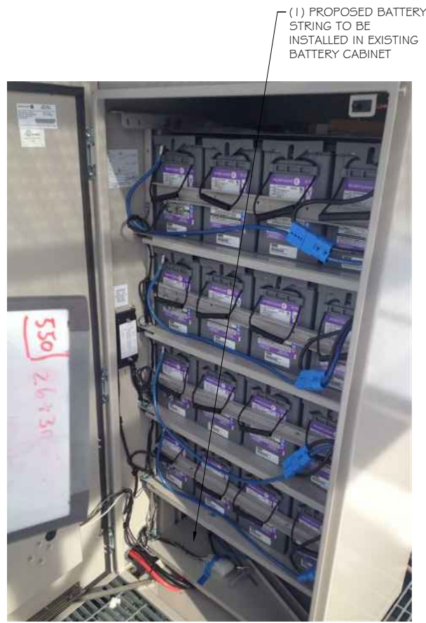
EXISTING BBU CABINET ③ SCALE: NTS
