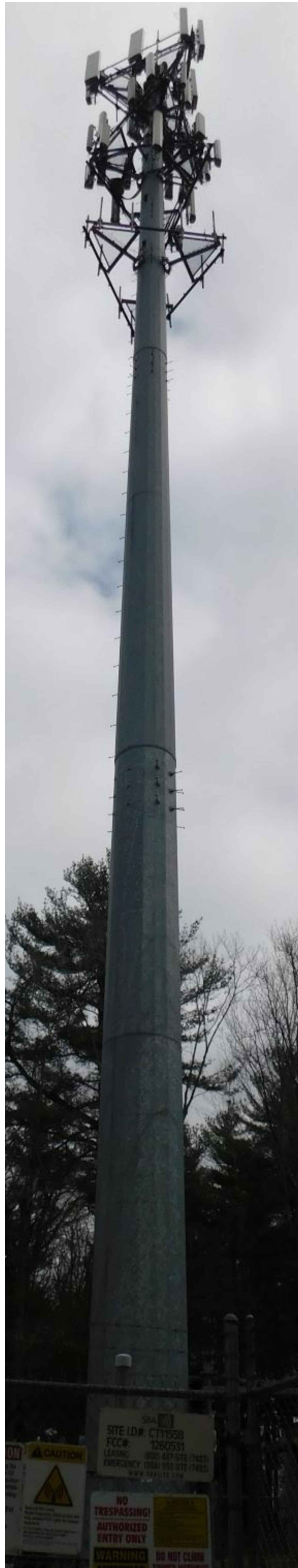
EXISTING ELEVATION PHOTO DETAIL
