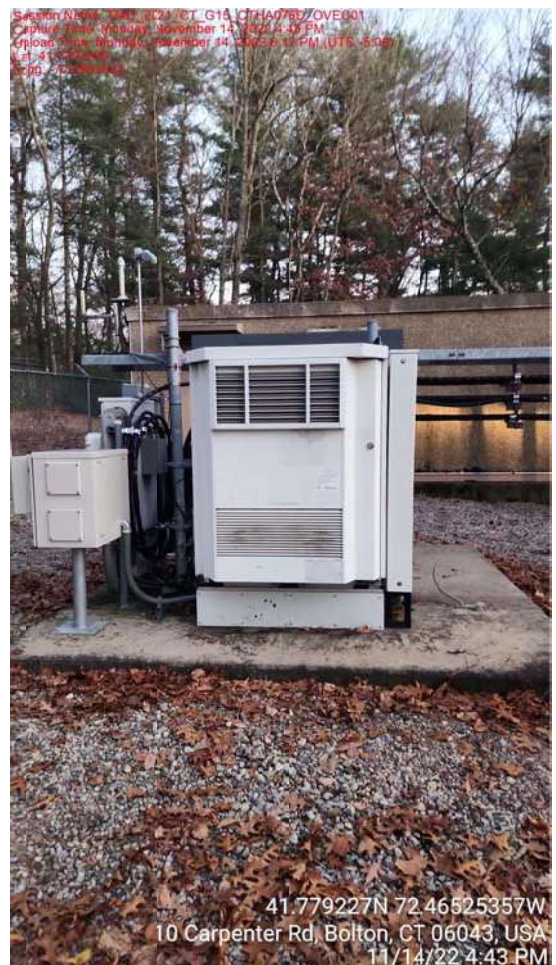
T-Mobile Ground Level Equipment Mounted To Existing Concrete Pad
