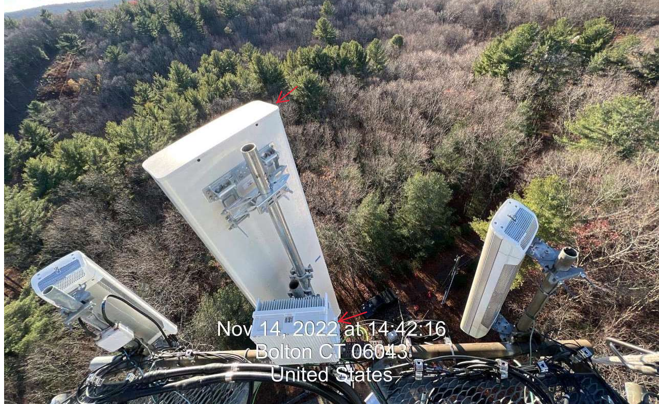
Gamma Sector: (1) New Antenna & (1) New RRH Mounted To Existing Low-Profile Platform
