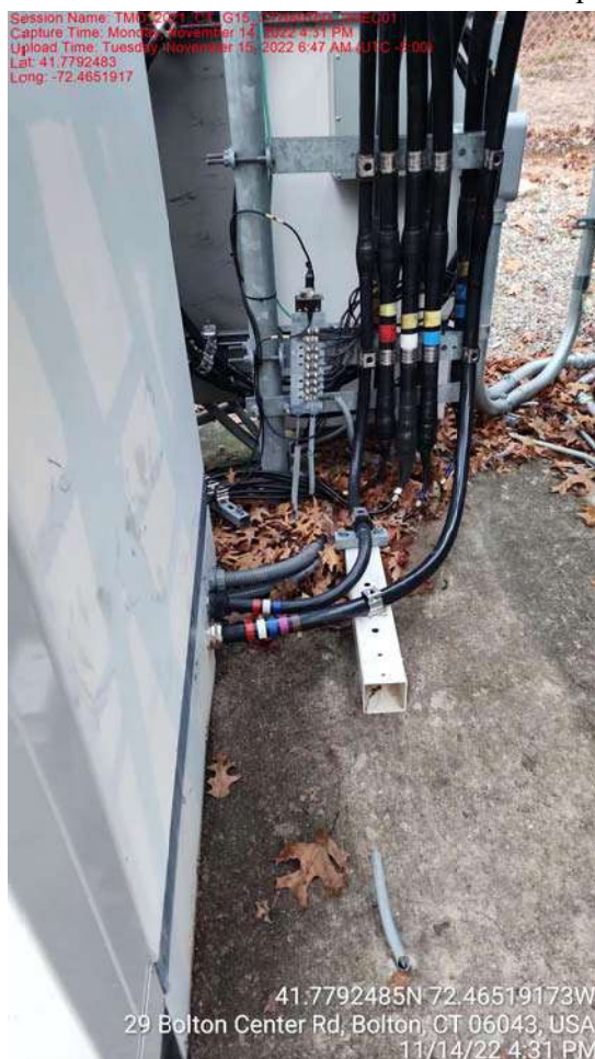
New Signal Cable At Existing Cabinet Run Along Existing Path
