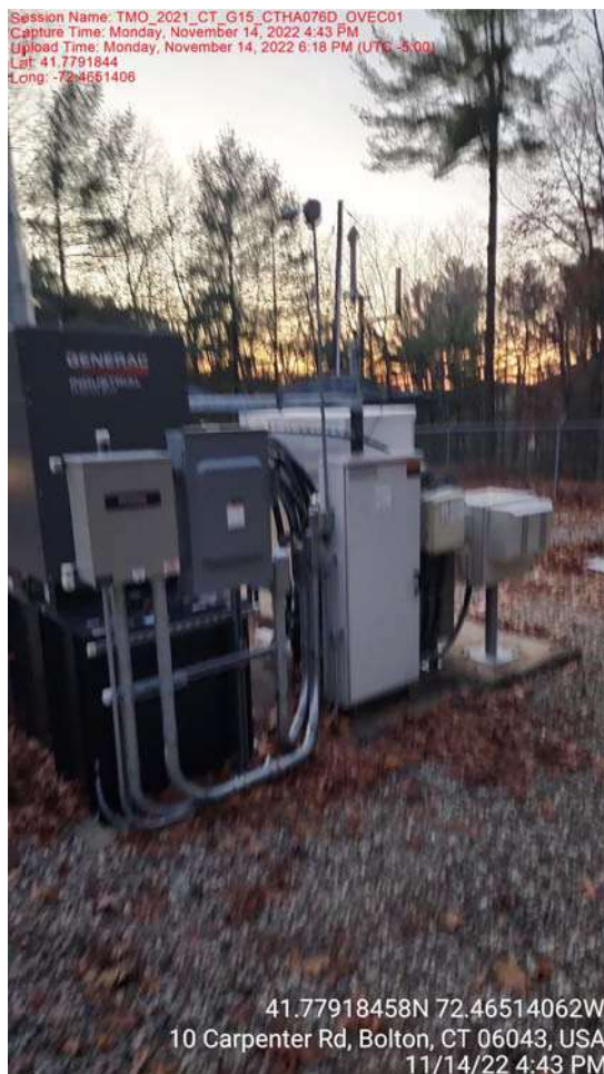
T-Mobile Ground Level Equipment Mounted To Existing Concrete Pad
