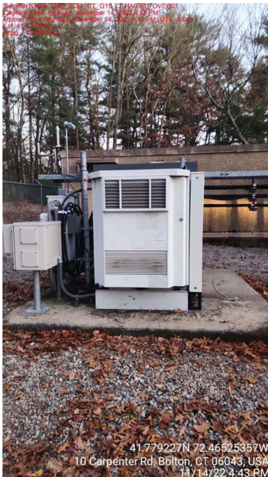
Existing Cabinet Mounted To Existing Concrete Pad
