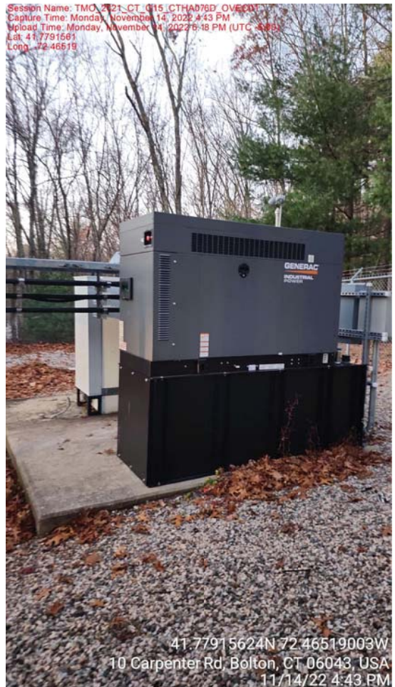
Existing Generator Mounted To Existing Concrete Pad
