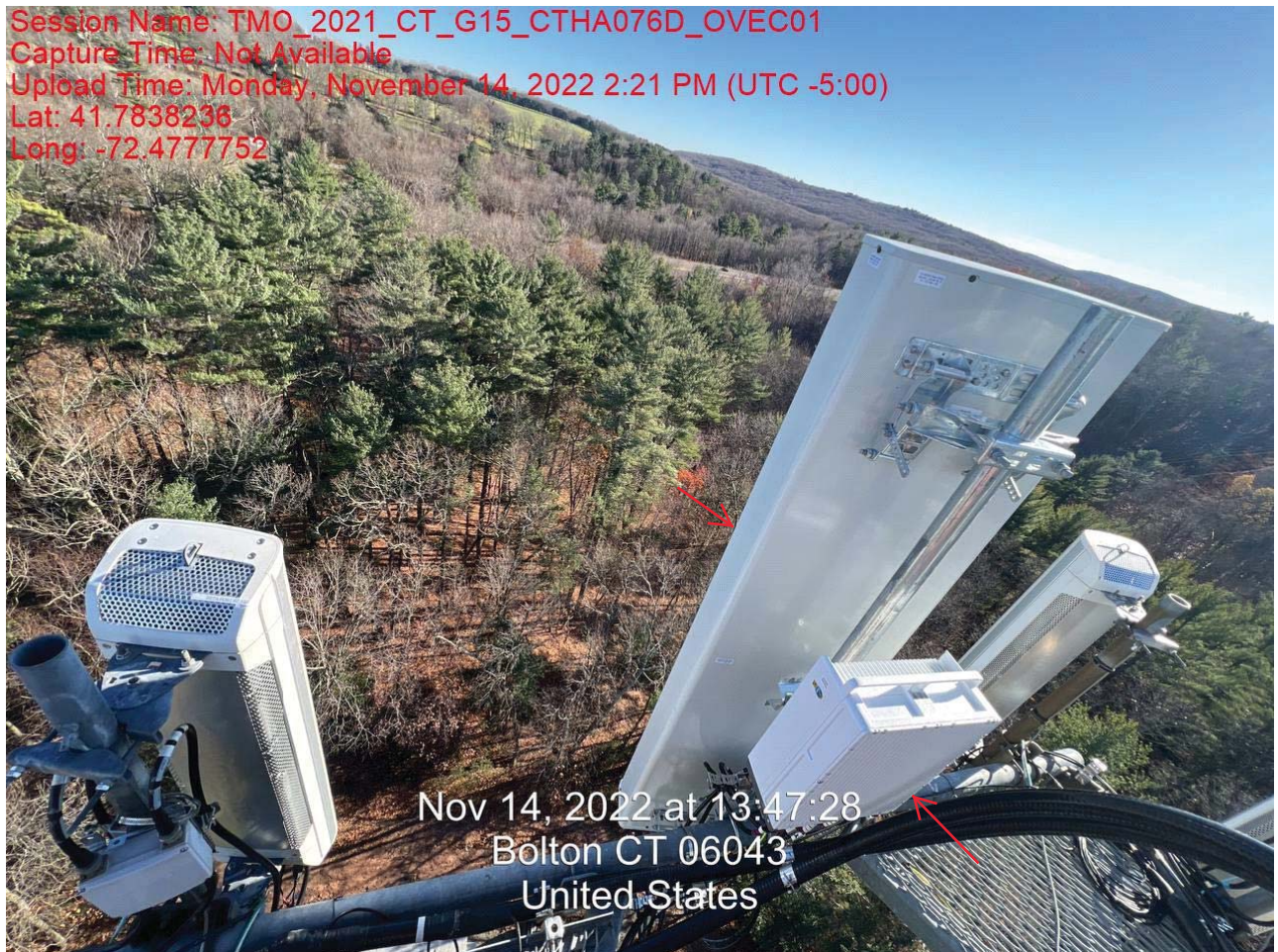
Beta Sector: (1) New Antenna & (1) New RRH Mounted To Existing Platform On Existing Monopole
