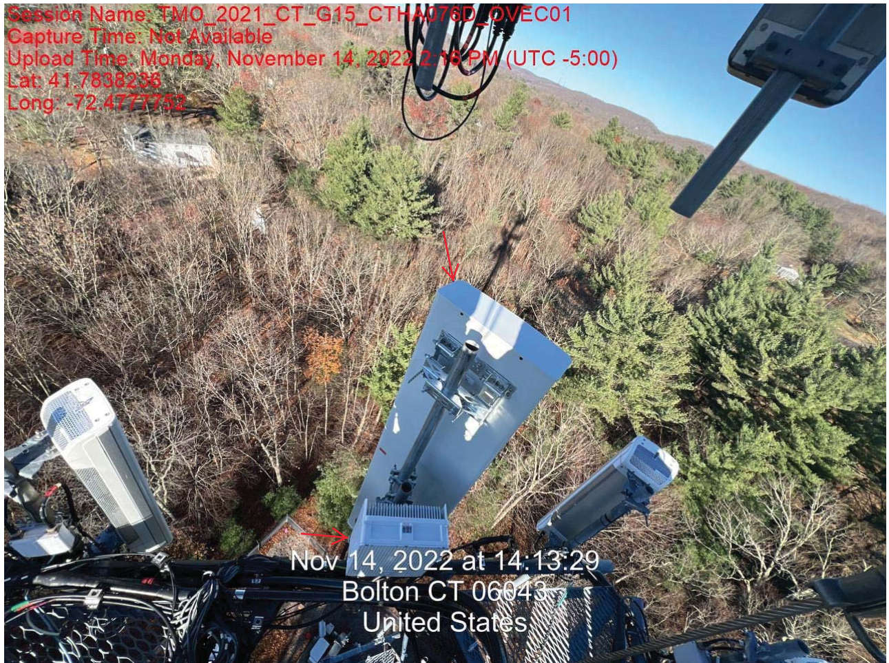
Alpha Sector: (1) New Antenna & (1) New RRH Mounted To Existing Platform On Existing Monopole
