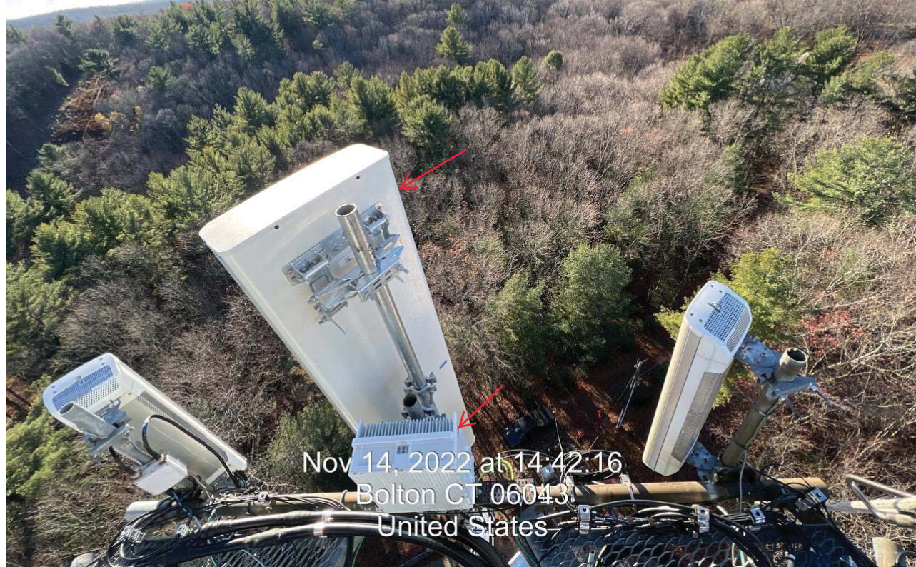
Gamma Sector: (1) New Antenna & (1) New RRH Mounted To Existing Platform On Existing Monopole
