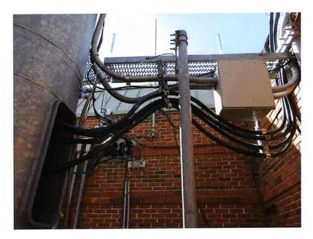
Photos of existing feed lines and ice bridges.
