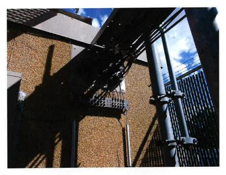
Photo of existing hatch plates and ground bar at shelter.
