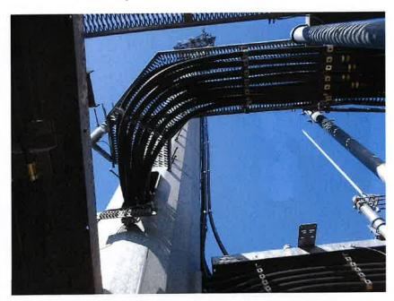
Photo of existing feed lines and ground bars at tower.
