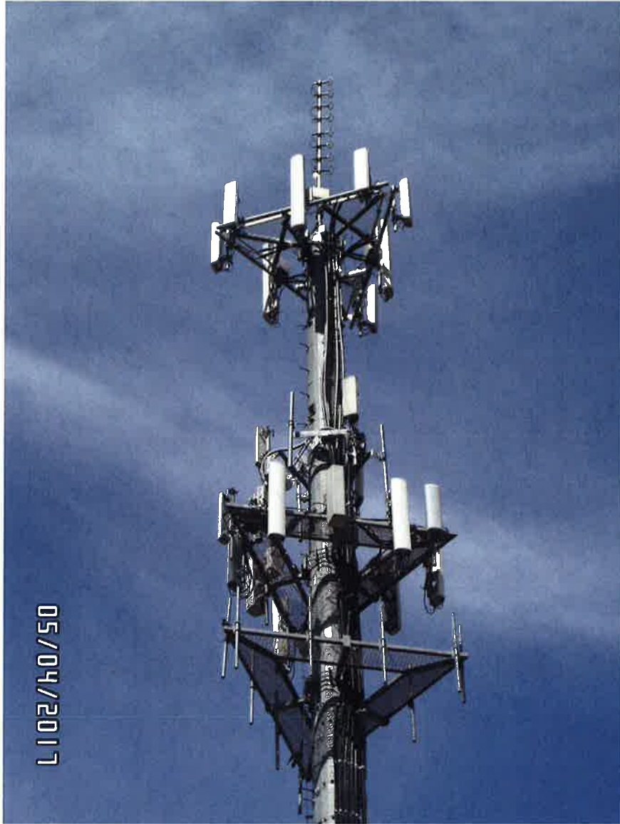
Photo 1: Photo illustrating the Monopole with Appurtenances shown.
