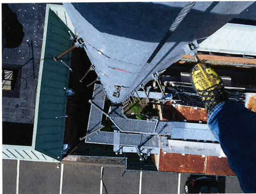
Overview photos of existing ice bridges from tower.
