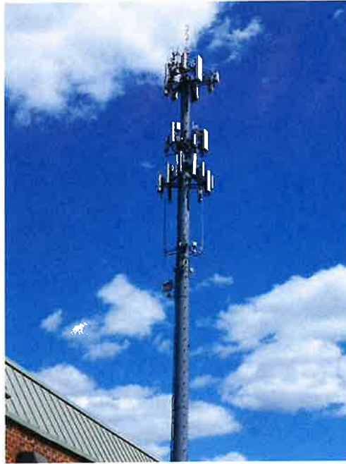
Overview photo of the existing 136' monopole tower.
