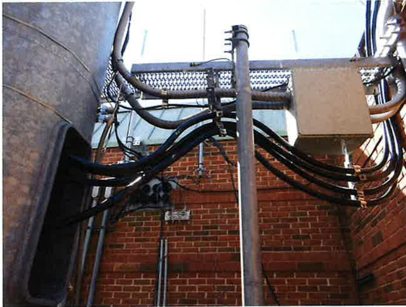
Photos of existing feed lines and ice bridges.
