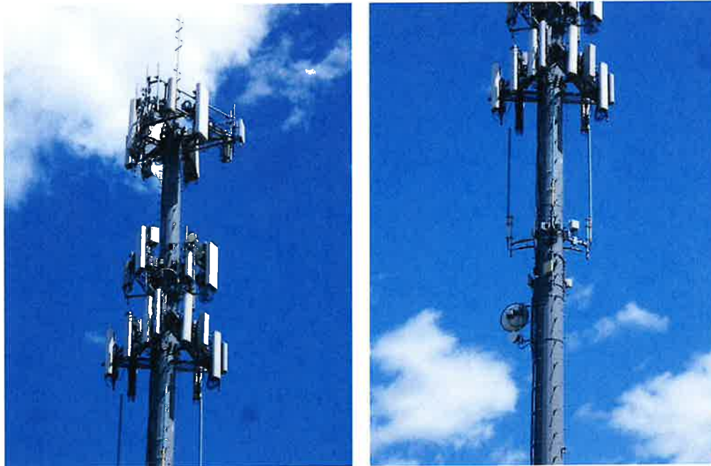
Overview photos of existing equipment and mounts.
