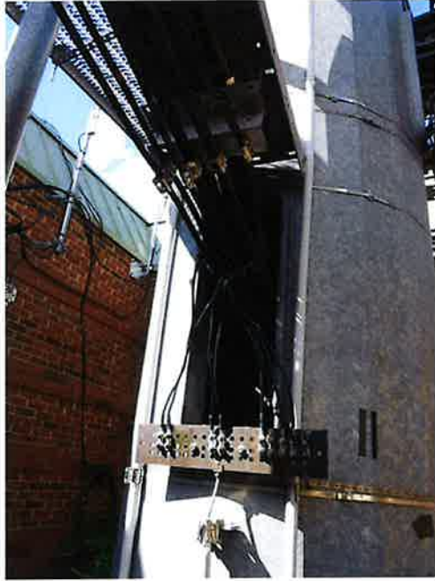
Additional photos of existing feed lines and ground bars at tower.
