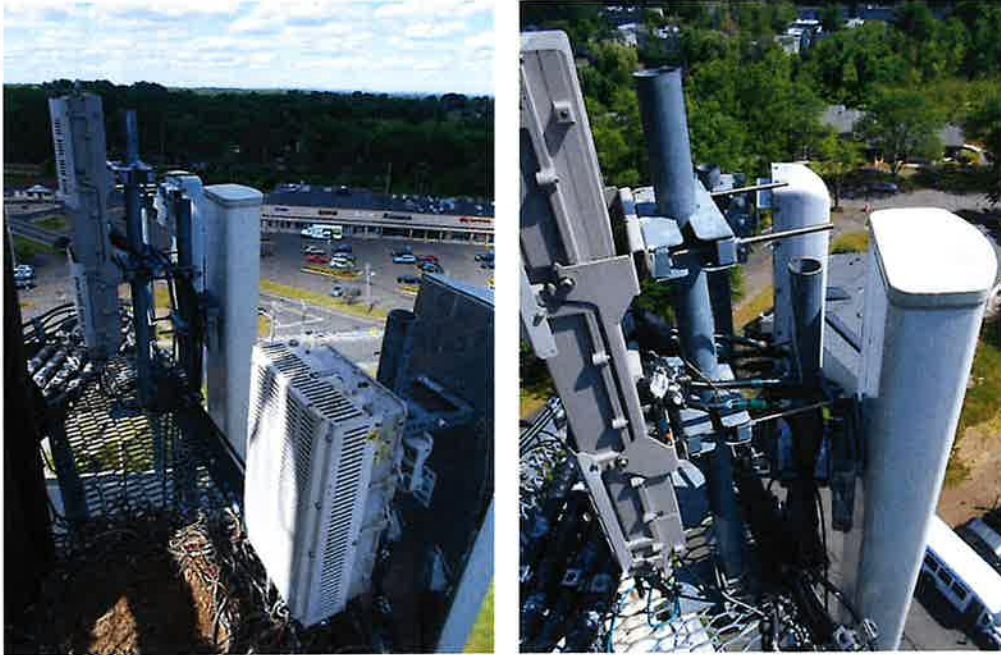
Photos of Verizon Wireless's typical existing equipment and mounts at 105'.
