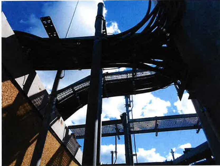
Photos of existing feed lines and ice bridges.
