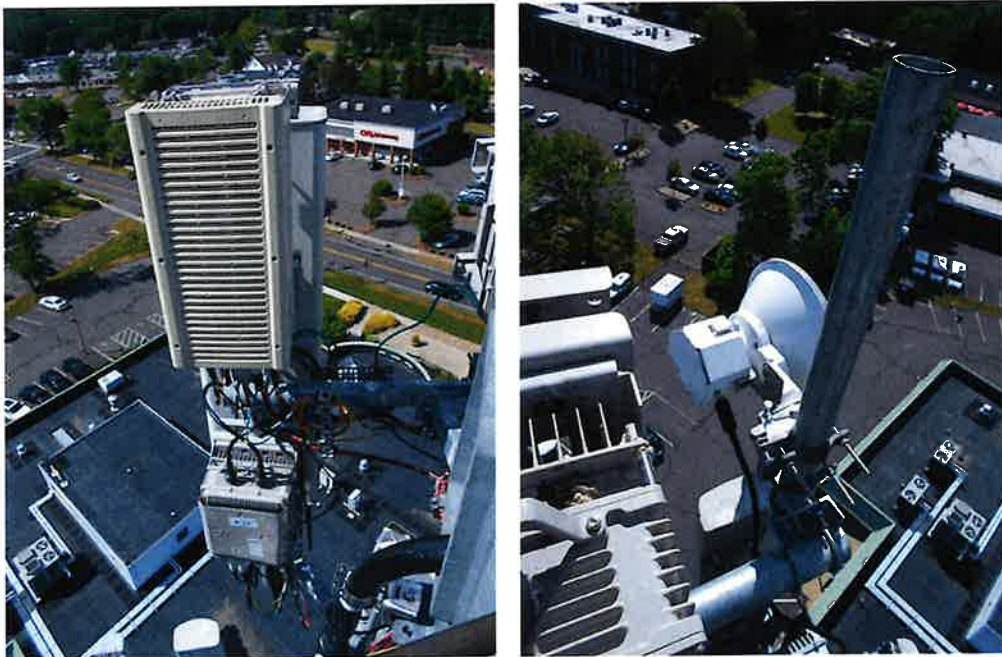
Additional photos of Sprint's typical existing equipment and mounts at 115'.
