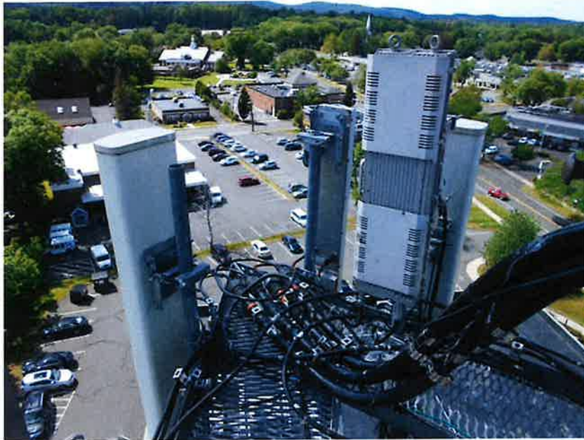
Additional photos of Verizon Wireless's typical existing equipment and mounts at 105'.
