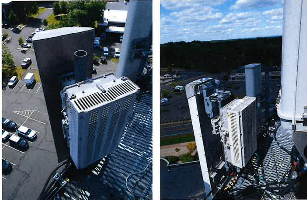
Additional photos of Verizon Wireless's typical existing equipment and mounts at 105'.
