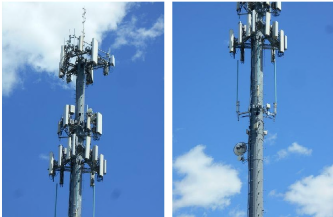
Overview photos of existing equipment and mounts.
