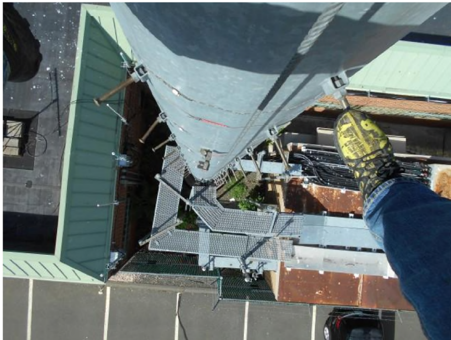
Overview photos of existing ice bridges from tower.
