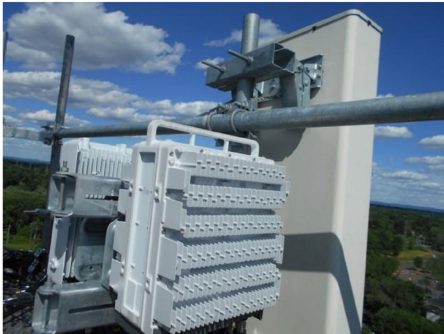
Additional photos of T-Mobile's typical existing equipment and mounts at 136'.
