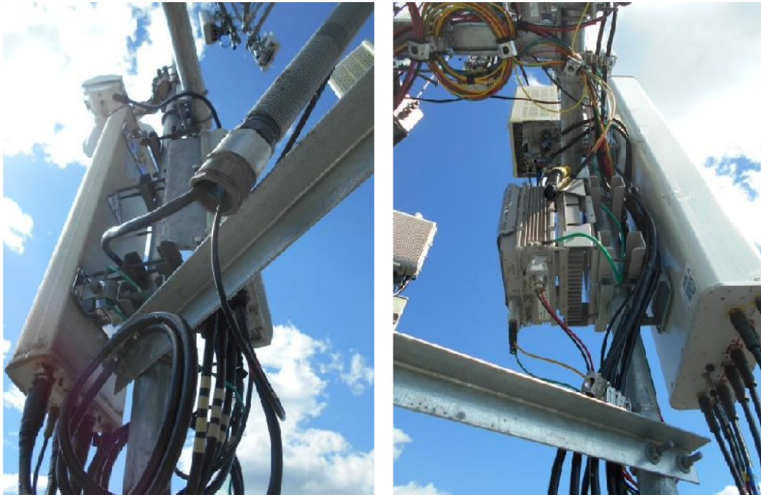
Photos of Sprint's typical existing equipment and mounts at 115'.
