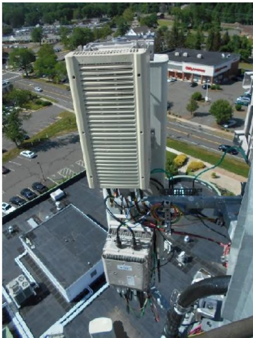
Additional photos of Sprint's typical existing equipment and mounts at 115'.
