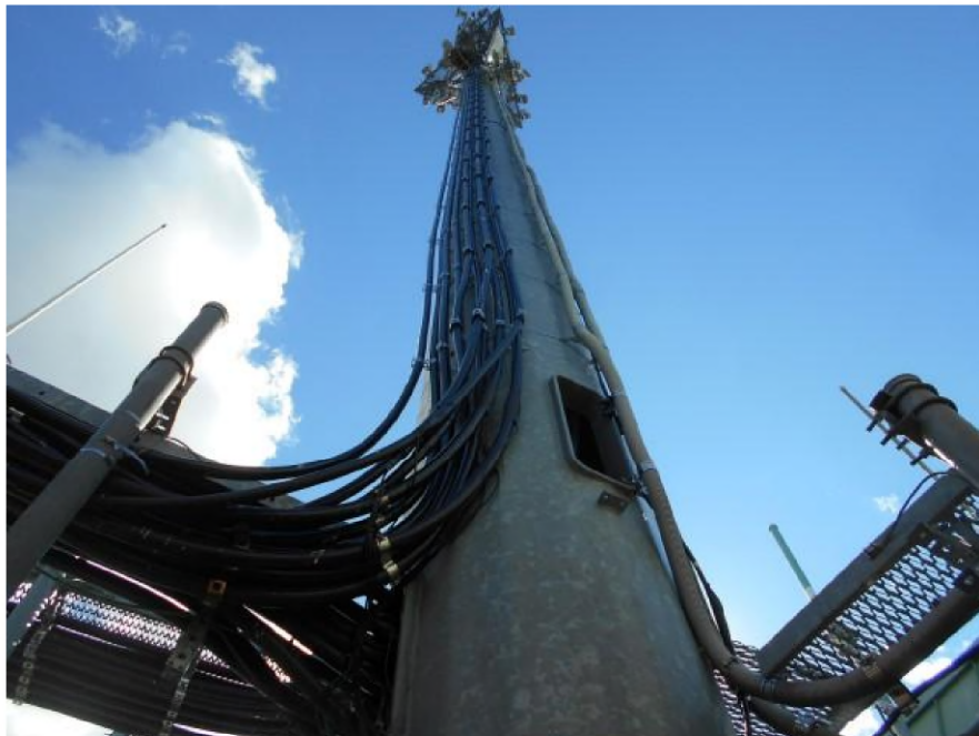
Additional photos of existing feed lines and ground bars at tower.
