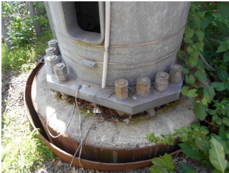
Photos of typical existing base foundation.
