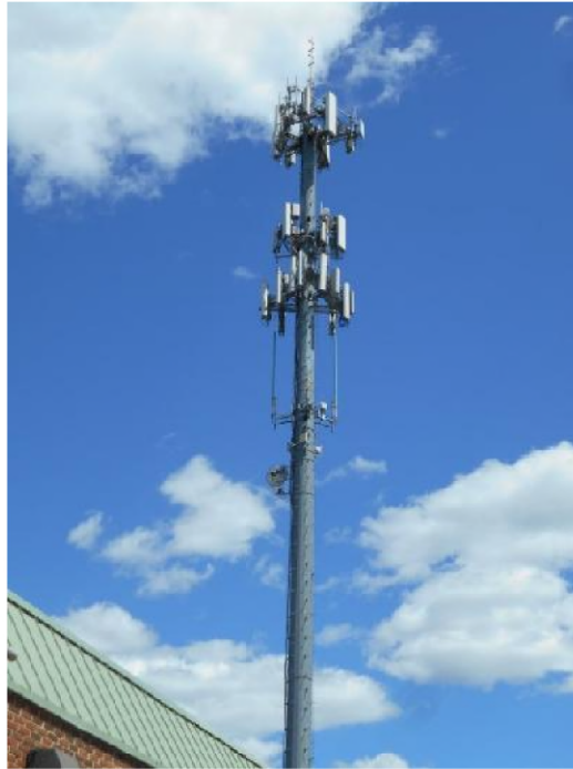
Overview photo of the existing 136' monopole tower.
