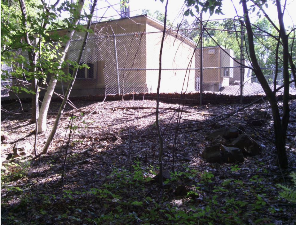
Northwest corner of compound. Compound would be expanded towards rocks in photo.
