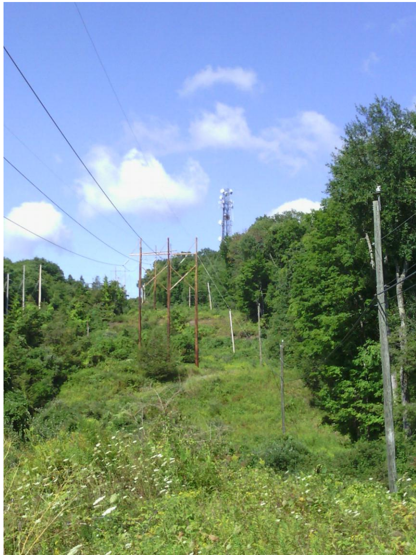
Existing tower from CL&P right-of-way, view west.
