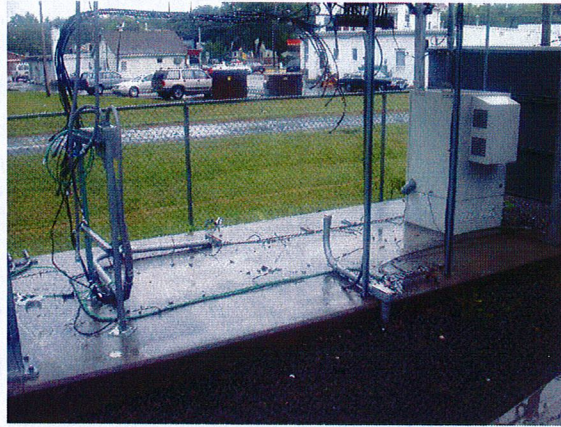
FORMER AT&T EQUIPMENT PAD TO BE CLEARED
