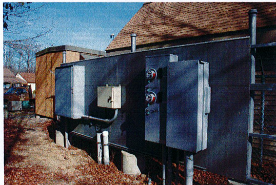
FORMER AT&T AC/TELEPHONE EQUIPMENT CLEARED
