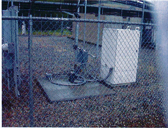
FORMER AT&T EQUIPMENT PAD TO BE CLEARED
