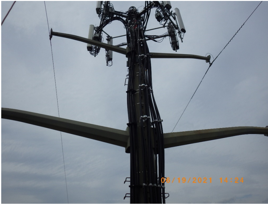
Photo - 5: Installation of feedlines
