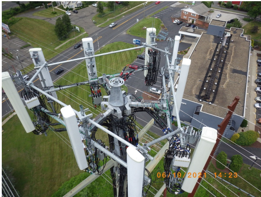
Photo - 4: Installation of antenna & remote radio heads, all positions
