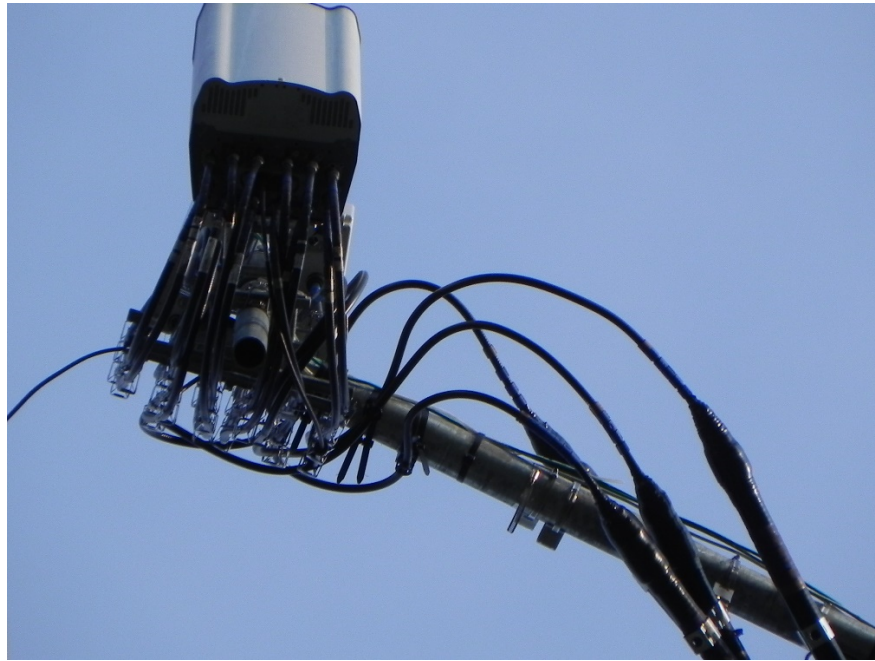
Photo - 3: Installation of antenna & remote radio heads, Position 3, Alpha Sector
