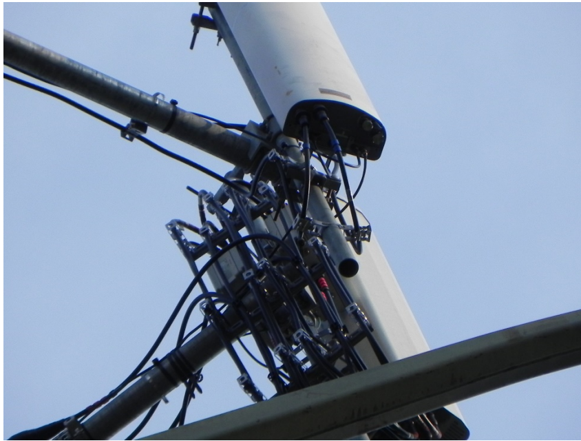
Photo - 1: Installation of antenna & remote radio heads, Position 1, Alpha Sector
