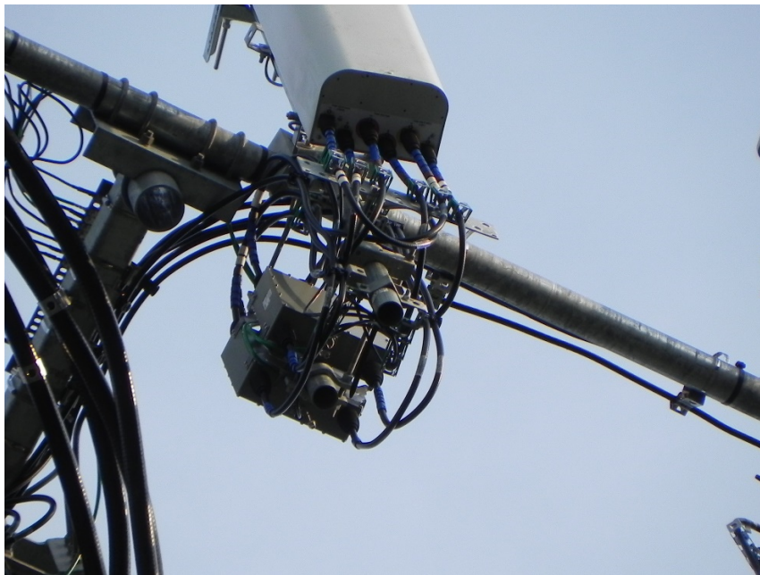
Photo - 2: Installation of antenna & remote radio heads, Position 2, Alpha Sector
