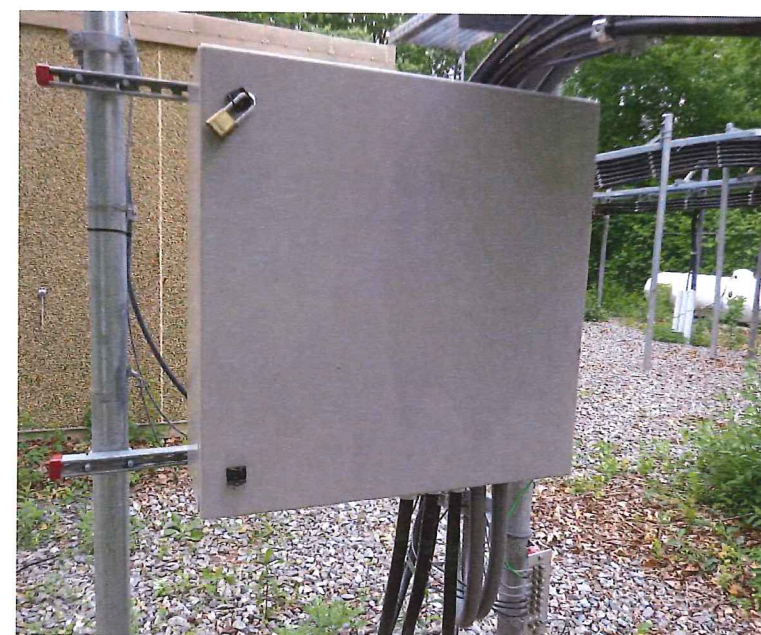
4 EXIST FIBER DISTRIBUTION BOX A-3 SCALE: NTS
