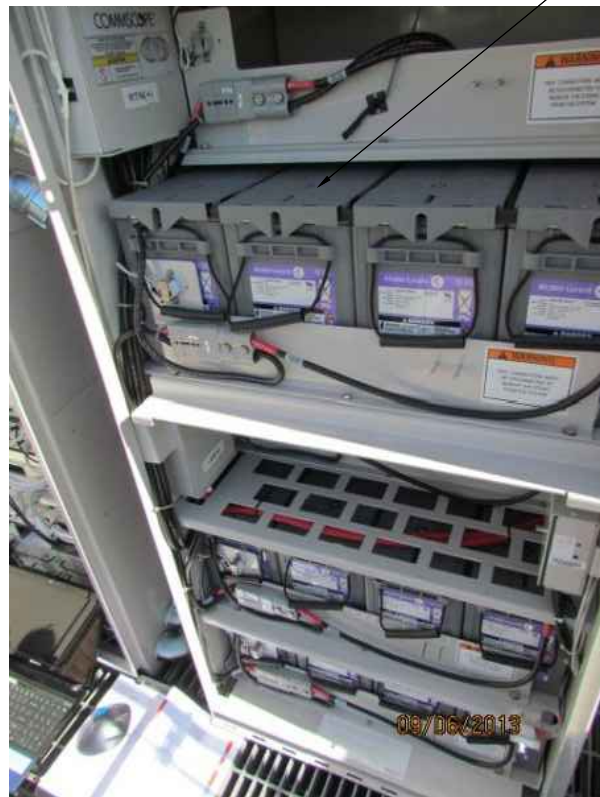
EXISTING BBU CABINET SCALE: NTS
