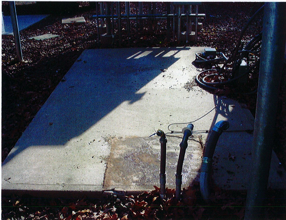
Pad after equipment removal
