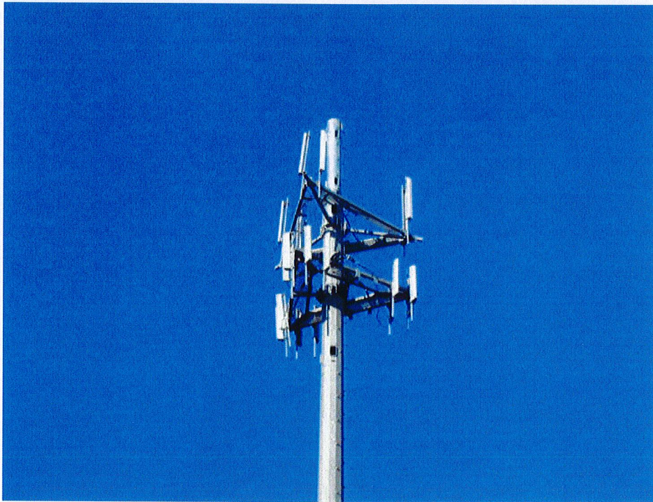
AT&T antenna array removed
