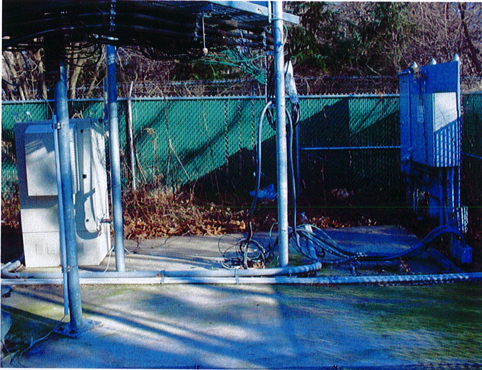
Cabinet and associated equipment before removal
