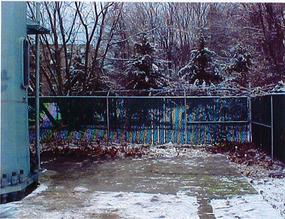
Cabinet and associated equipment after removal
