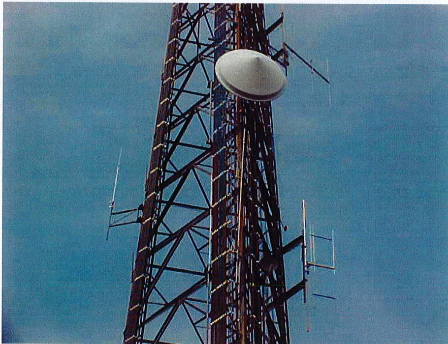
AT&T antenna array removed
