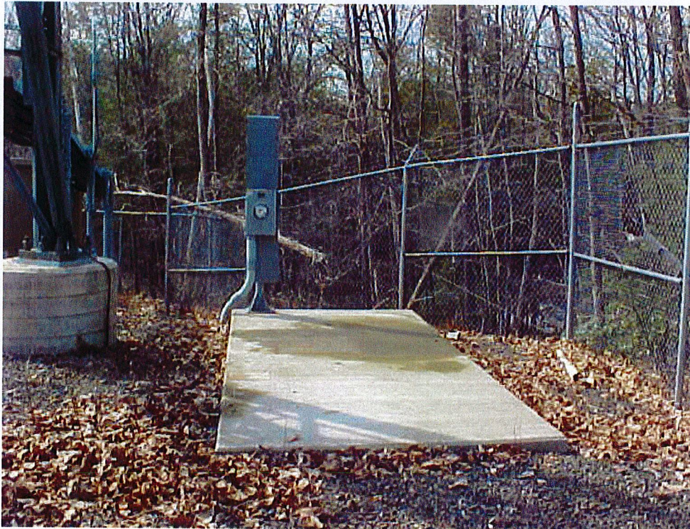
AT&T base station and associated equipment removed
