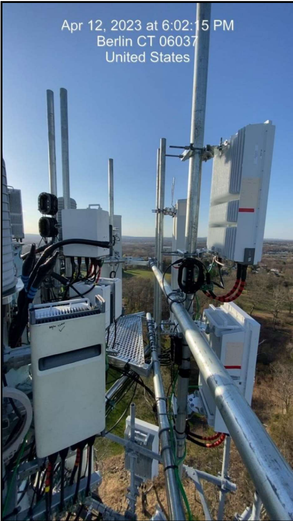
Figure 4: View(s) of installed RRUs and Squids on new mount platform
