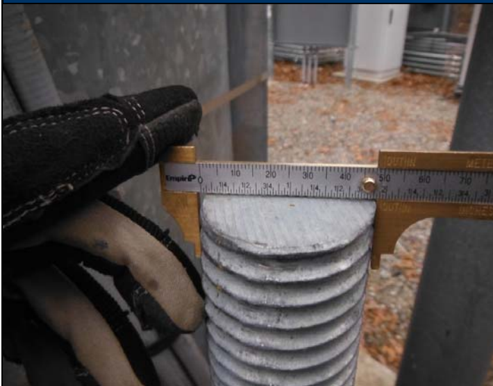
PH#15 Installation of Modification – Installation of New Anchor Rods
