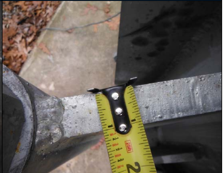
PH#20 Installation of Modification – Installation of Anchor Rod Transfer Sleeves
