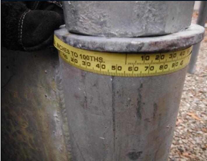
PH#23 Installation of Modification – Installation of Anchor Rod Transfer Sleeves
