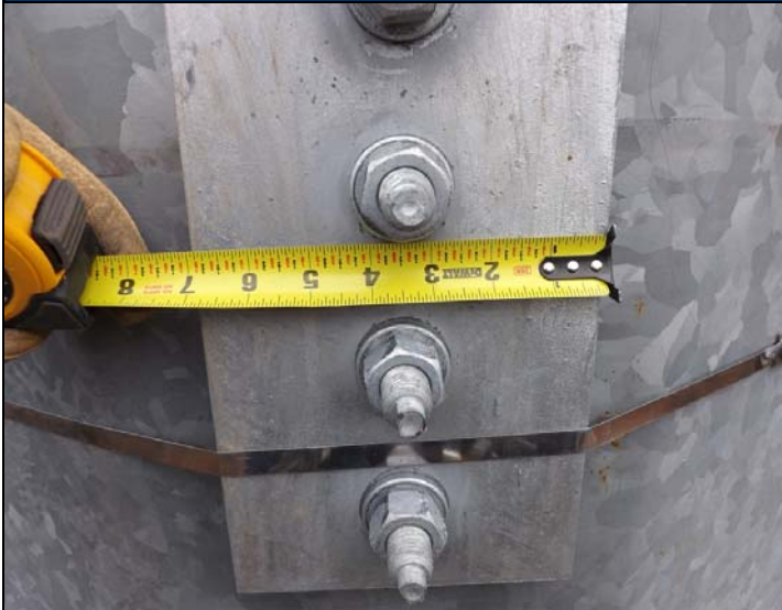
PH#07 Installation of Modification – Installation of Flat Plate Reinforcement
