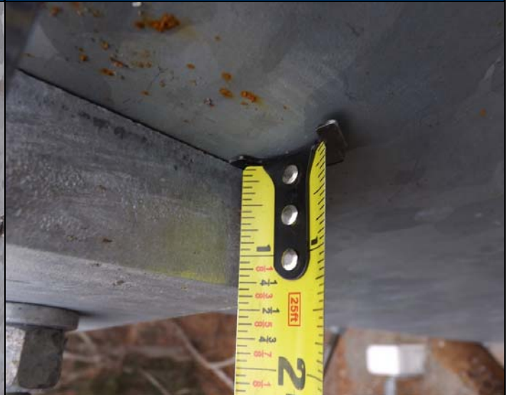
PH#08 Installation of Modification – Installation of Flat Plate Reinforcement
