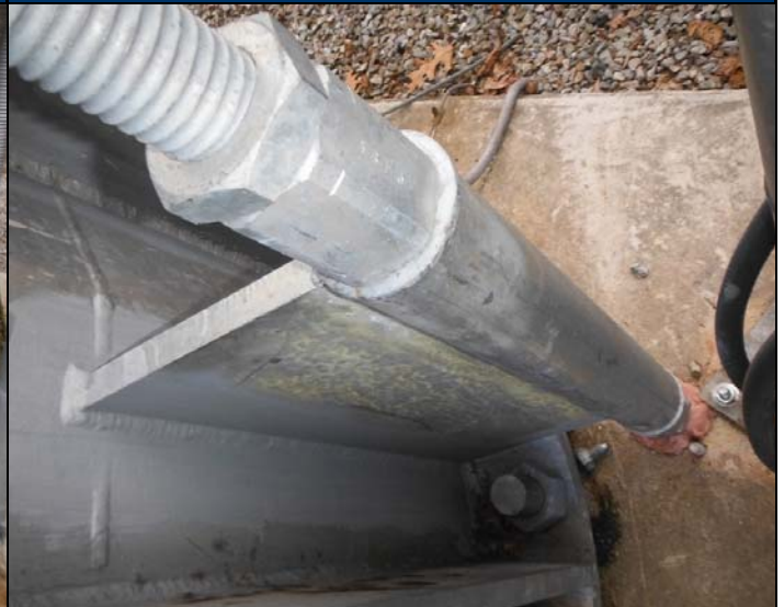
PH#12 Installation of Modification – Installation of New Anchor Rods
