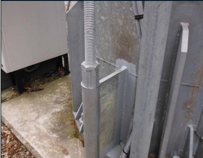
PH#15 Installation of Modification – Installation of New Anchor Rods
