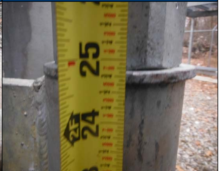
PH#24 Installation of Modification – Installation of Anchor Rod Transfer Sleeves
