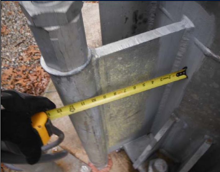
PH#19 Installation of Modification – Installation of Anchor Rod Transfer Sleeves
