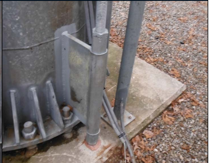
PH#16 Installation of Modification – Installation of New Anchor Rods
