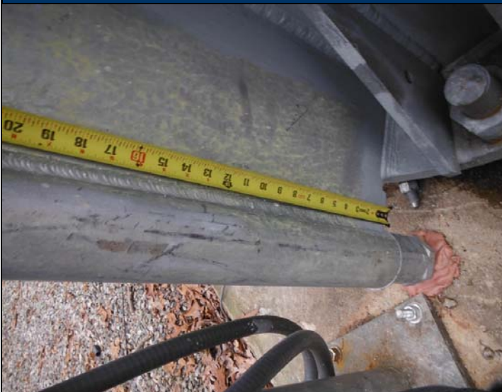
PH#19 Installation of Modification – Installation of Anchor Rod Transfer Sleeves
