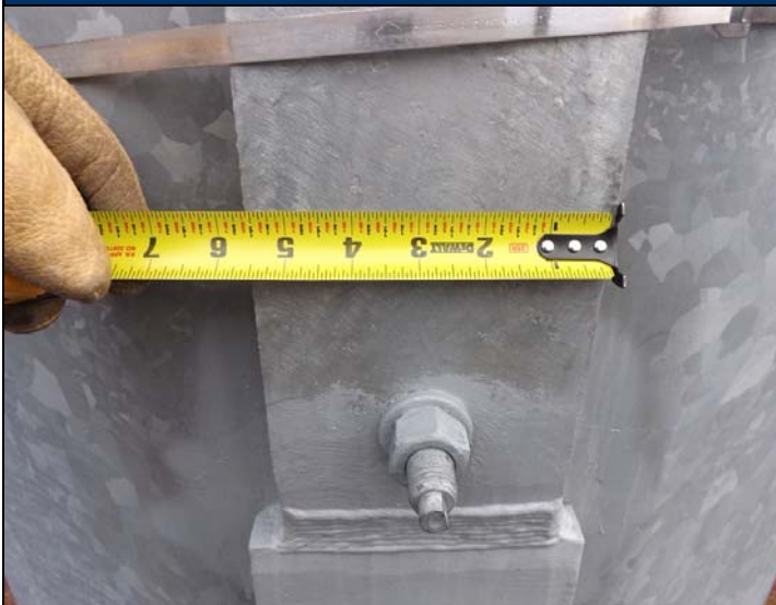
PH#07 Installation of Modification – Installation of Flat Plate Reinforcement
