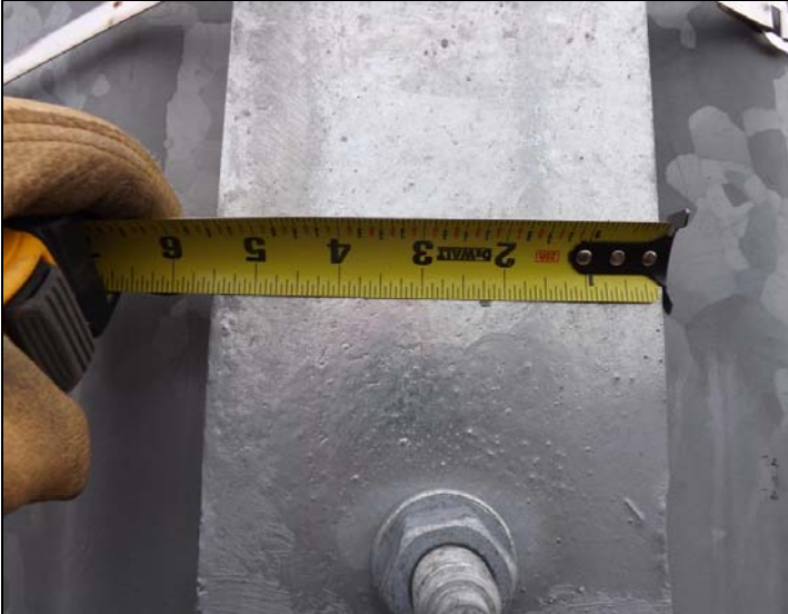
PH#11 Installation of Modification – Installation of New Anchor Rods
