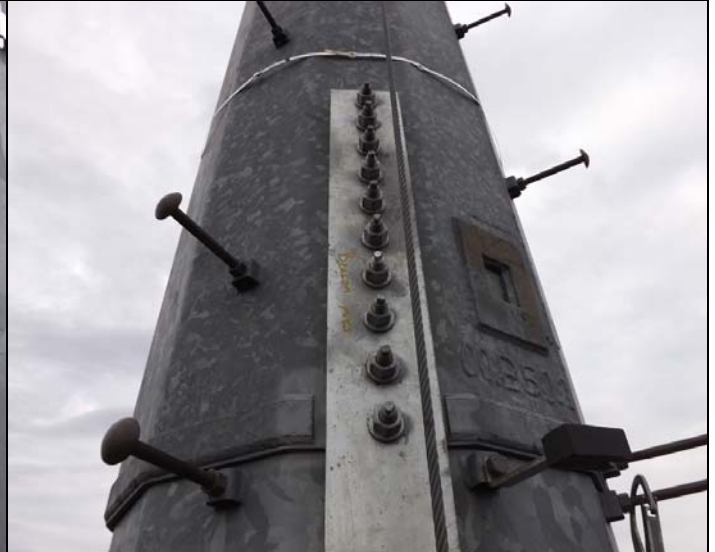
PH#12 Installation of Modification – Installation of New Anchor Rods
