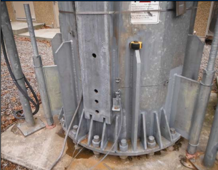
PH#11 Installation of Modification – Installation of New Anchor Rods
