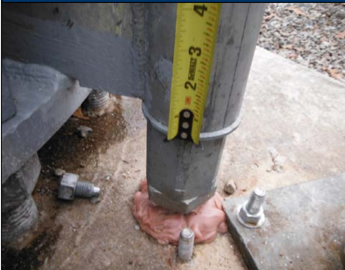
PH#23 Installation of Modification – Installation of Anchor Rod Transfer Sleeves
