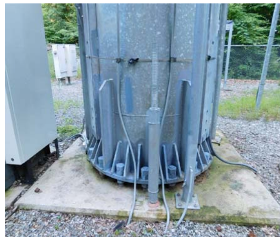
TOWER BASE/FOUNDATION PHOTO
