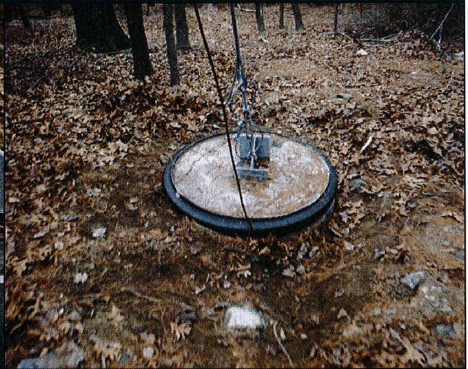
PH#12 Installation of Modification – Installation of Lug Plate
