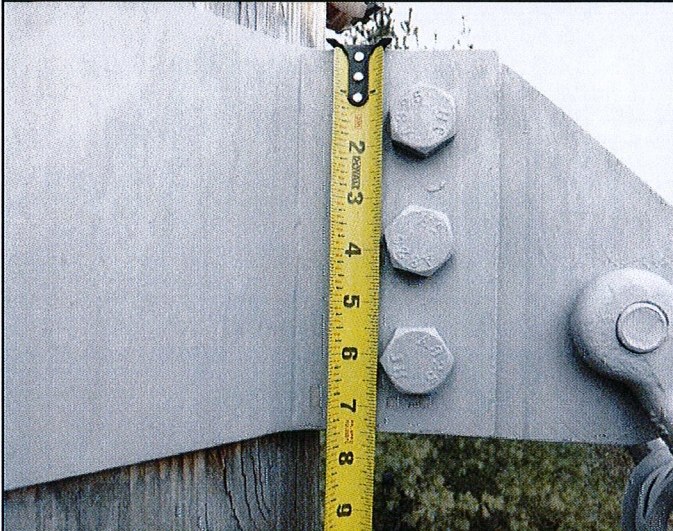
PH#15 Installation of Modification – Installation of Lug Plate
