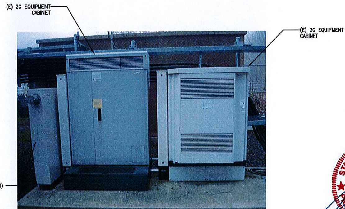
EXISTING EQUIPMENT AREA. N.T.S.
