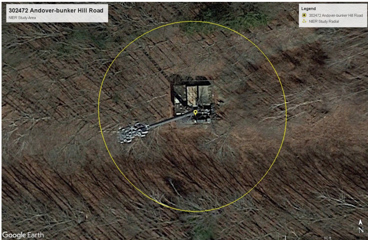
Aerial View of Site
