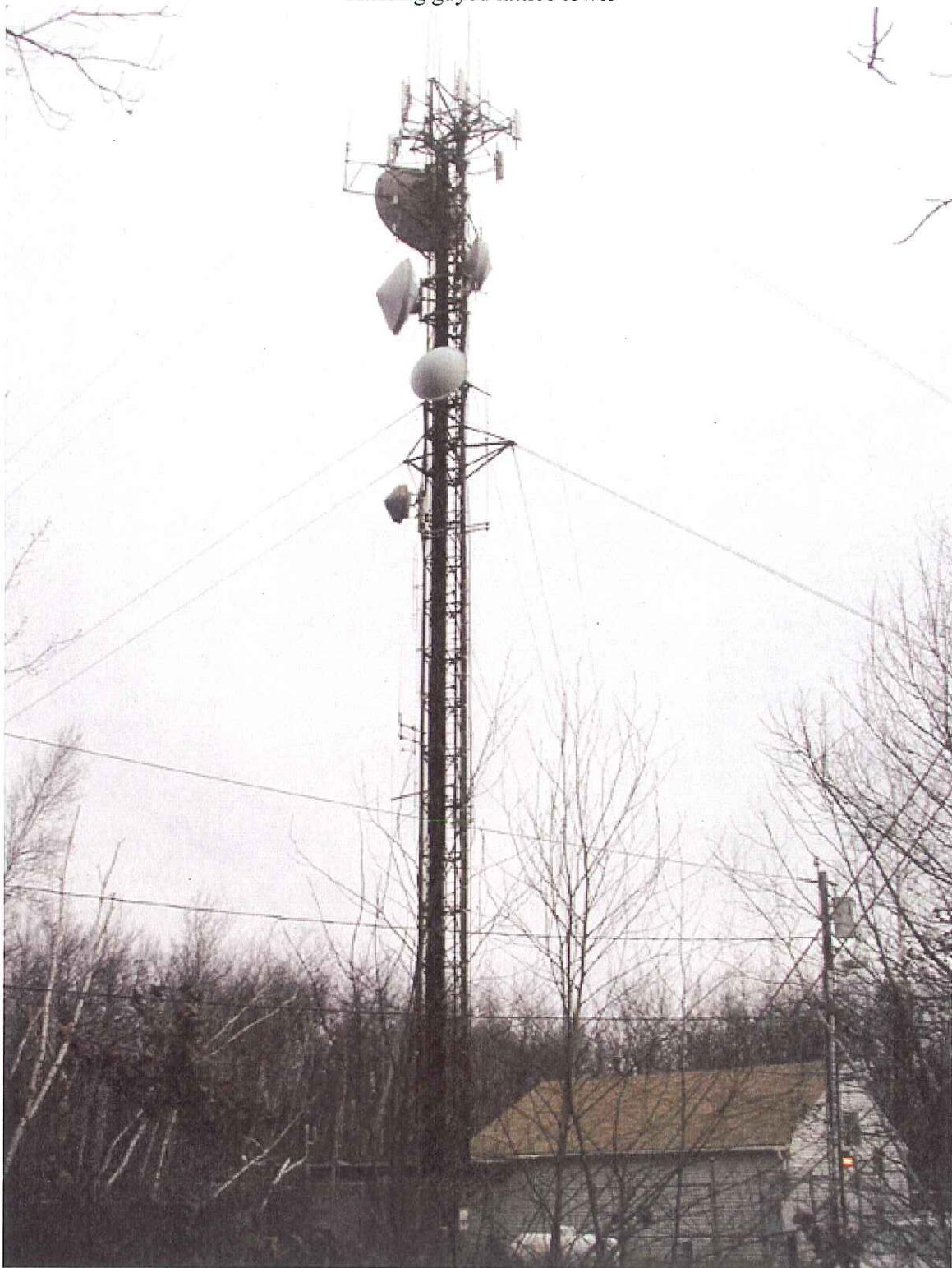
Existing guyed lattice tower
