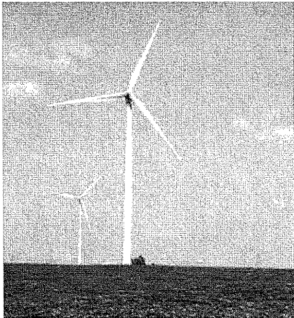
Utility-scale wind turbines located in Huron County, Michigan.
