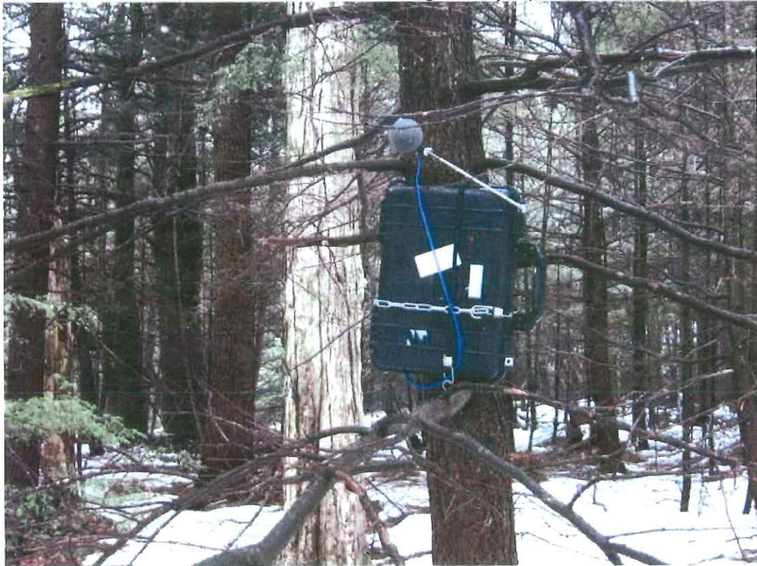
FIGURE 2: Installation Location for Site #1; Wagner Property, NW of Lake.
