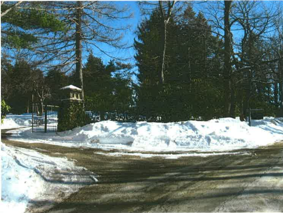
The gates into Rock Hall
