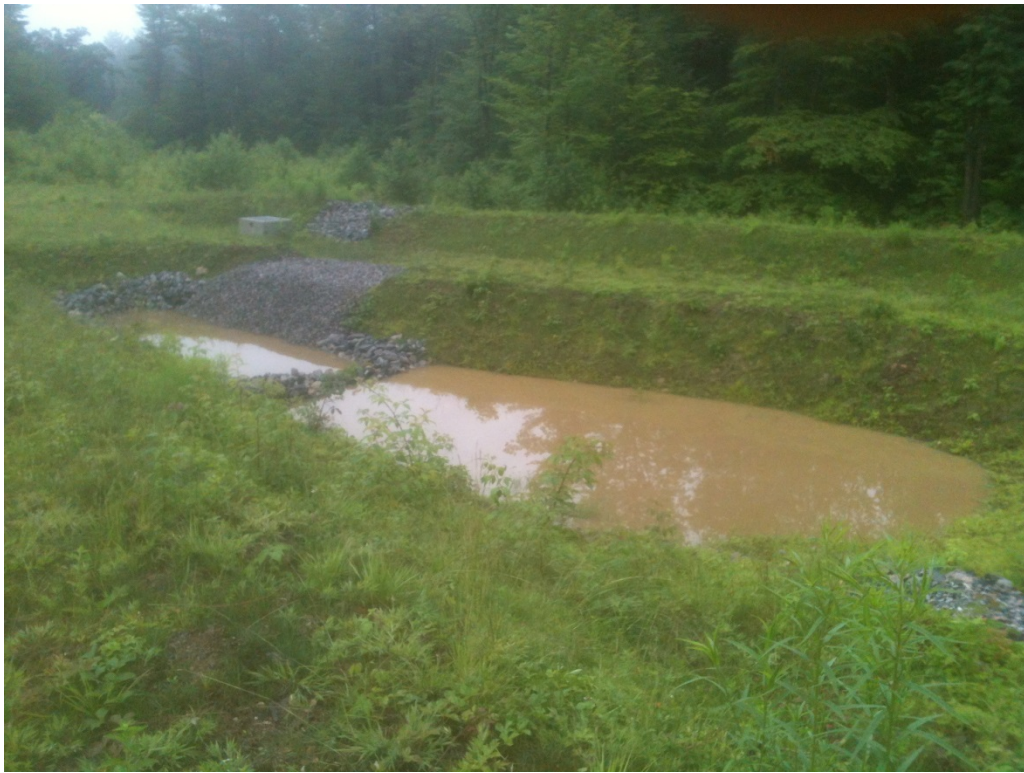
Temporary Sediment basin# 2, functioning as designed
