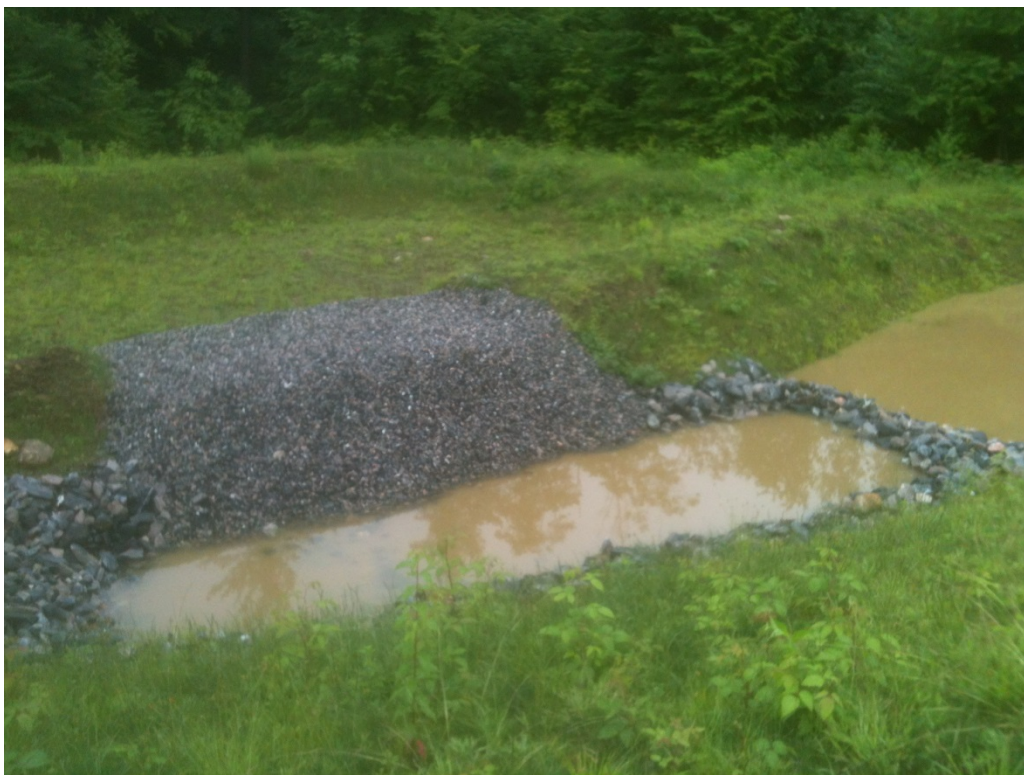
Temporary Sediment basin# 2, functioning as designed
