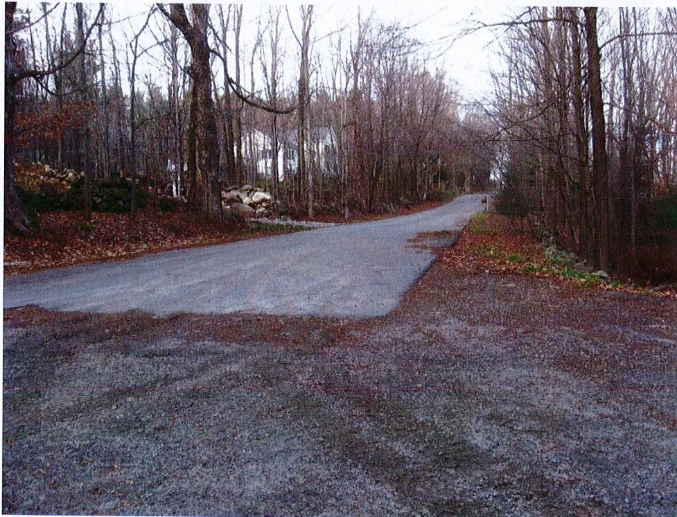
Flagg Hill Road – Gravel cul-de-sac at end of road
