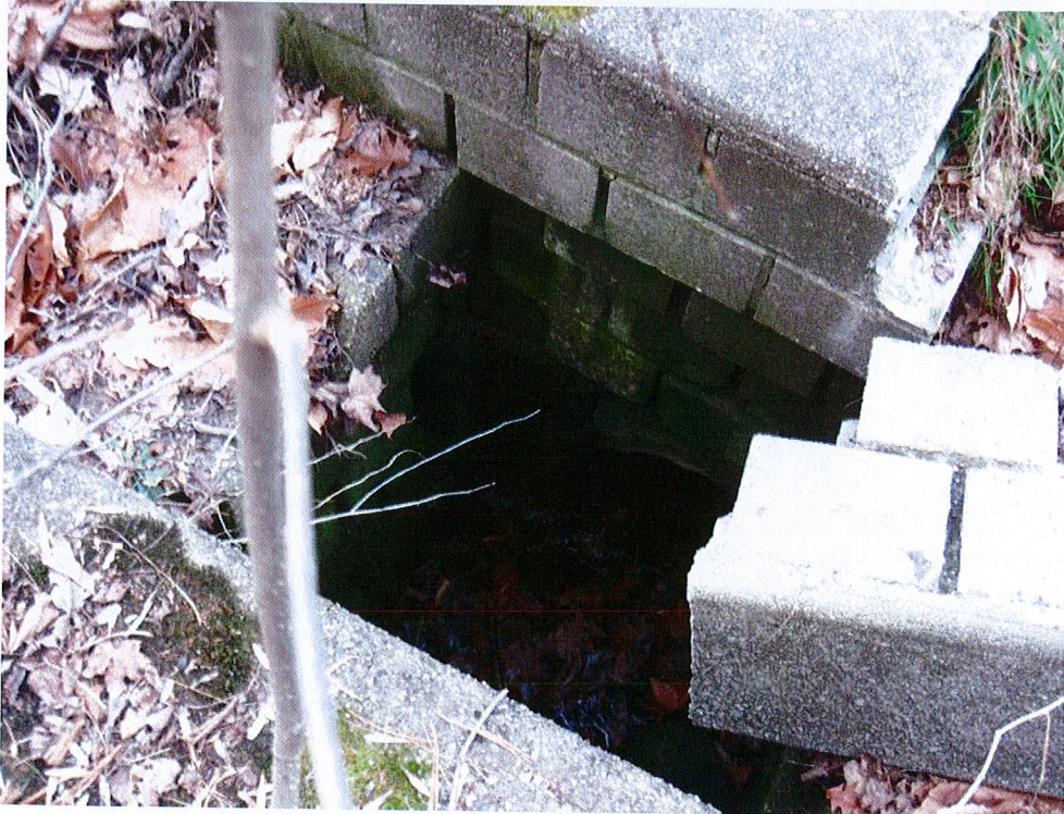
Flagg Hill Road – CMU catch basin structure and culvert, West Side
