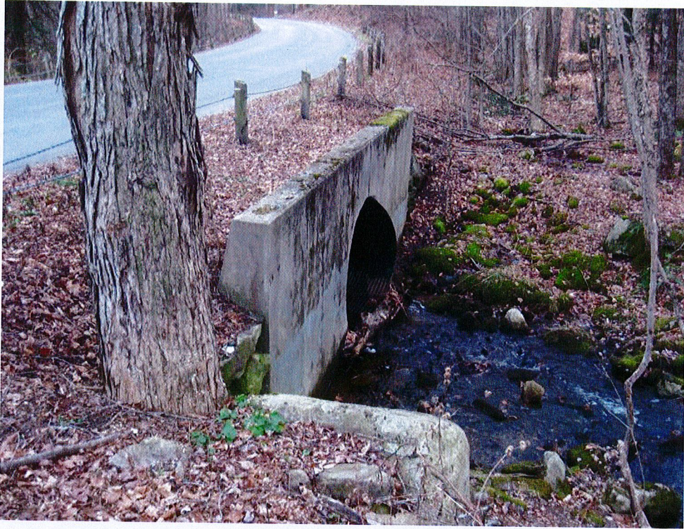
Flagg Hill Road – Culvert South of Route 44, West Side
