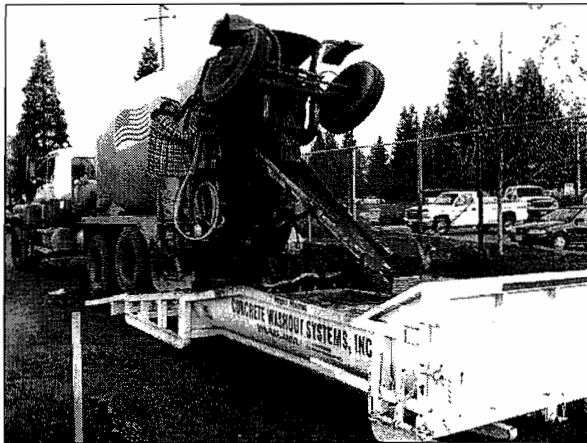
A concrete truck washing down his chute in a Concrete Washout Systems bin, which provides proper containment and method for capturing the wastewater and material.
