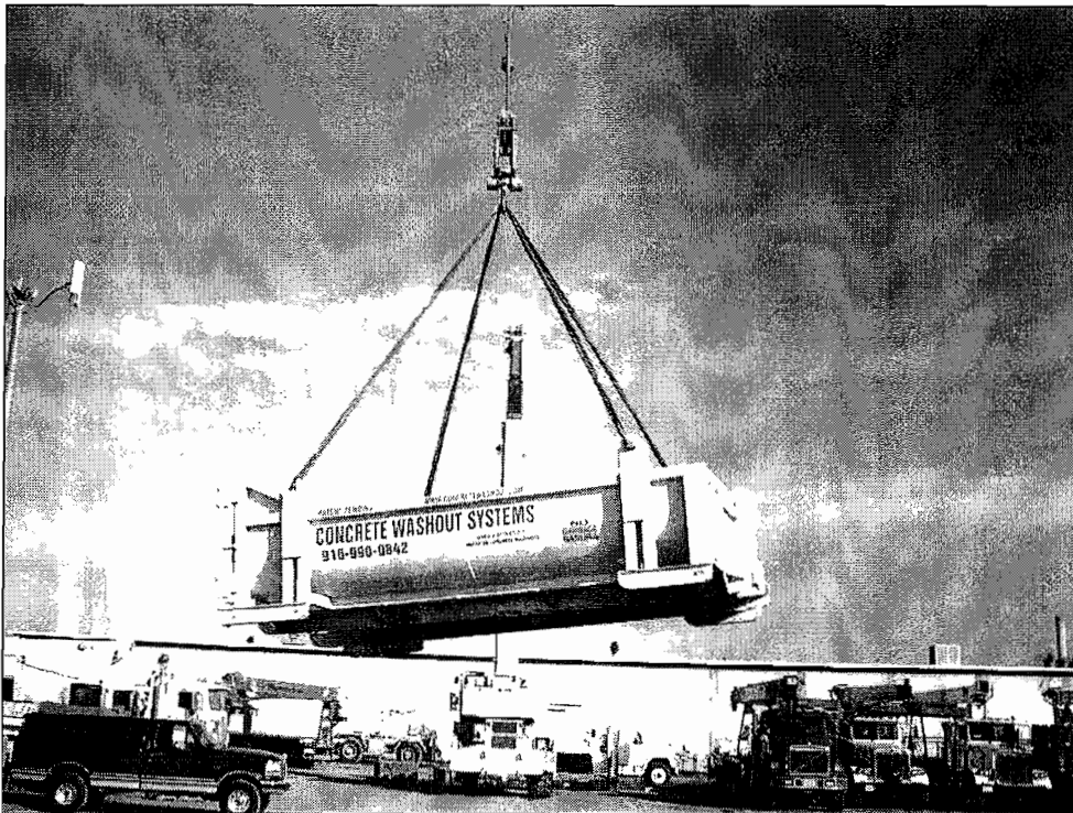
A rampless concrete washout systems container with hook points being craned.
