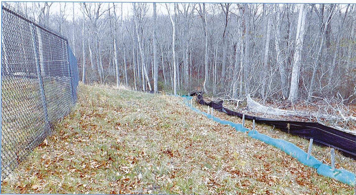
Southeast section of project site. Side slopes now stabilized with vegetation.
