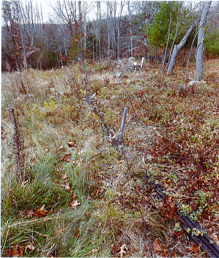
Silt fence adjacent Wingardner Property.
