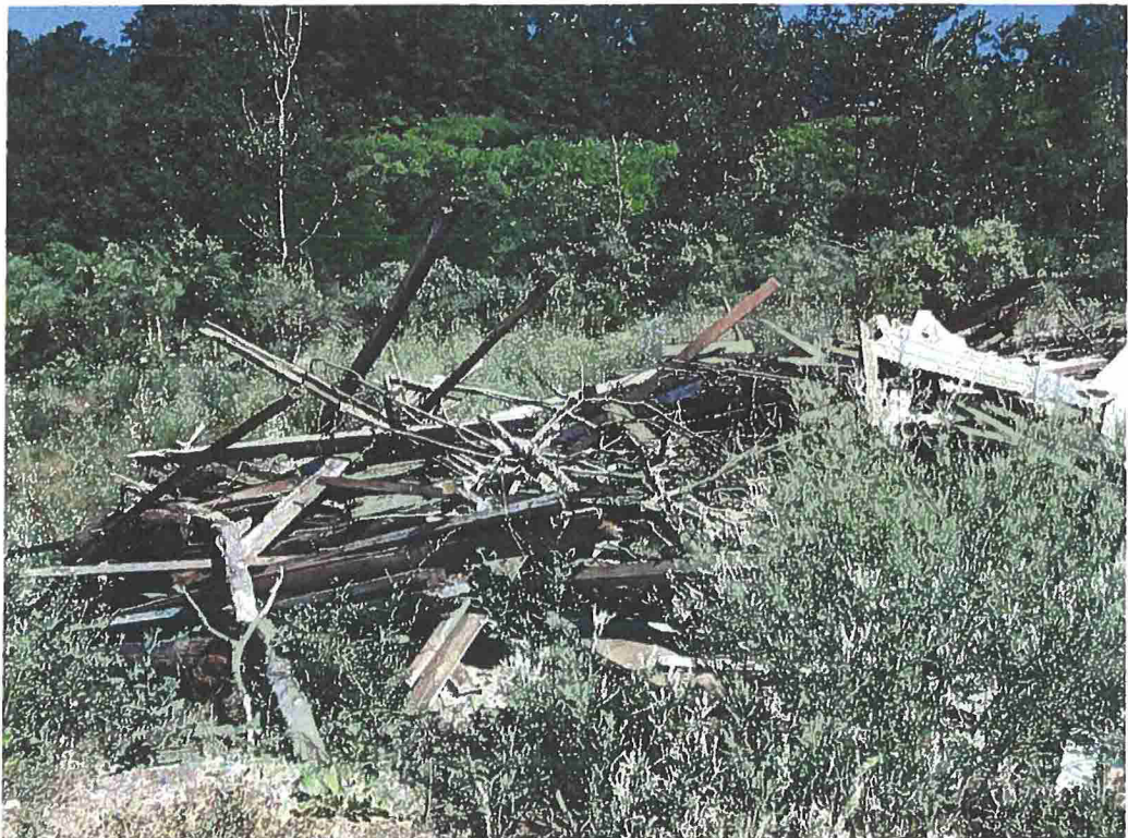
Wood debris, concrete, and asphalt piles observed on the northwest corner of the Site
