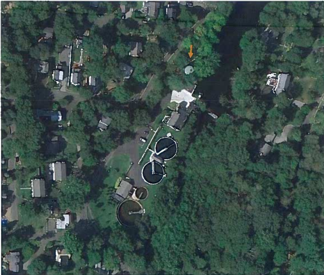
Figure 17 - Aerial View of Valley Road Water Treatment Facility, with Water Tank
