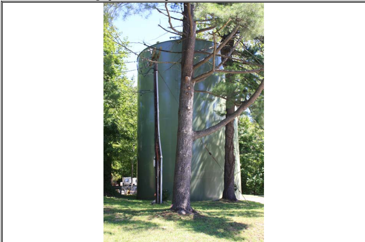
Photograph 2 - View looking northeast at existing water tank.
