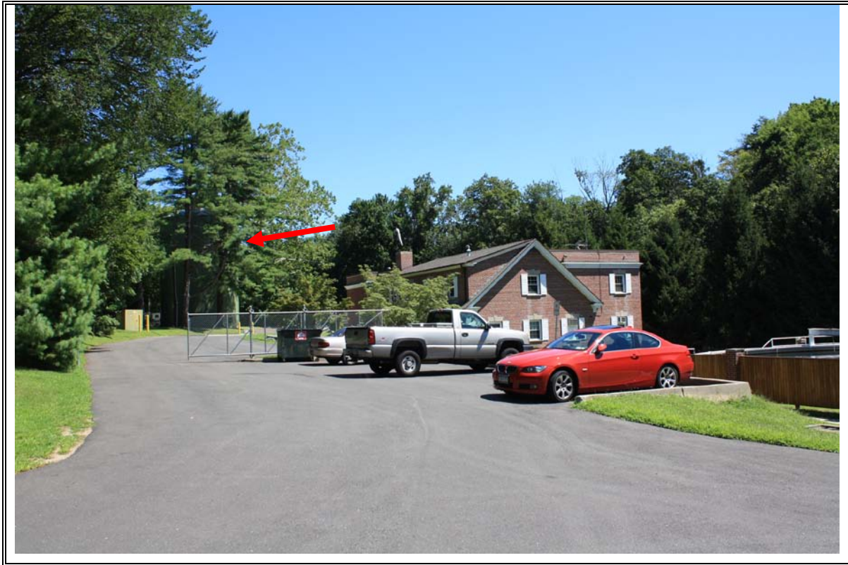
Photograph 1 – Existing water tank located behind trees.
