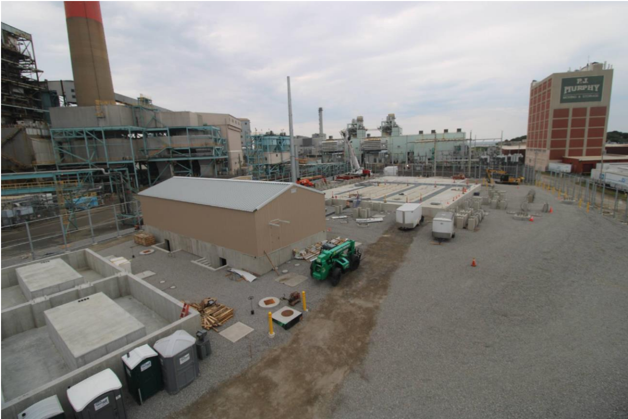
Photo 1: Broadview of project site with PDC Building being completed.
